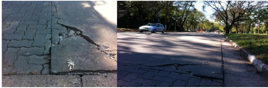
Figure 91. Distresses in the transition between interlock pavement and the short CRCP
