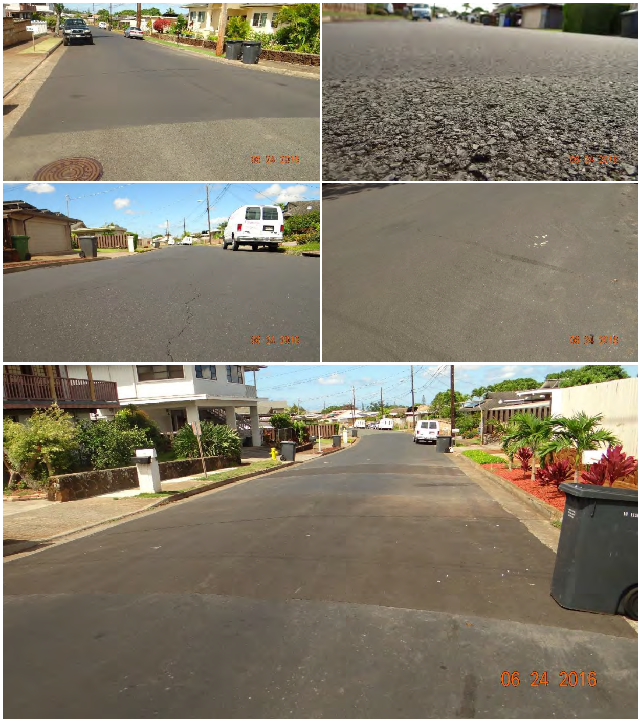
Figure C-71 Condition of Kaweloka Street section 3, treated with MasterSeal™ RTU, on 6/24/2016.
