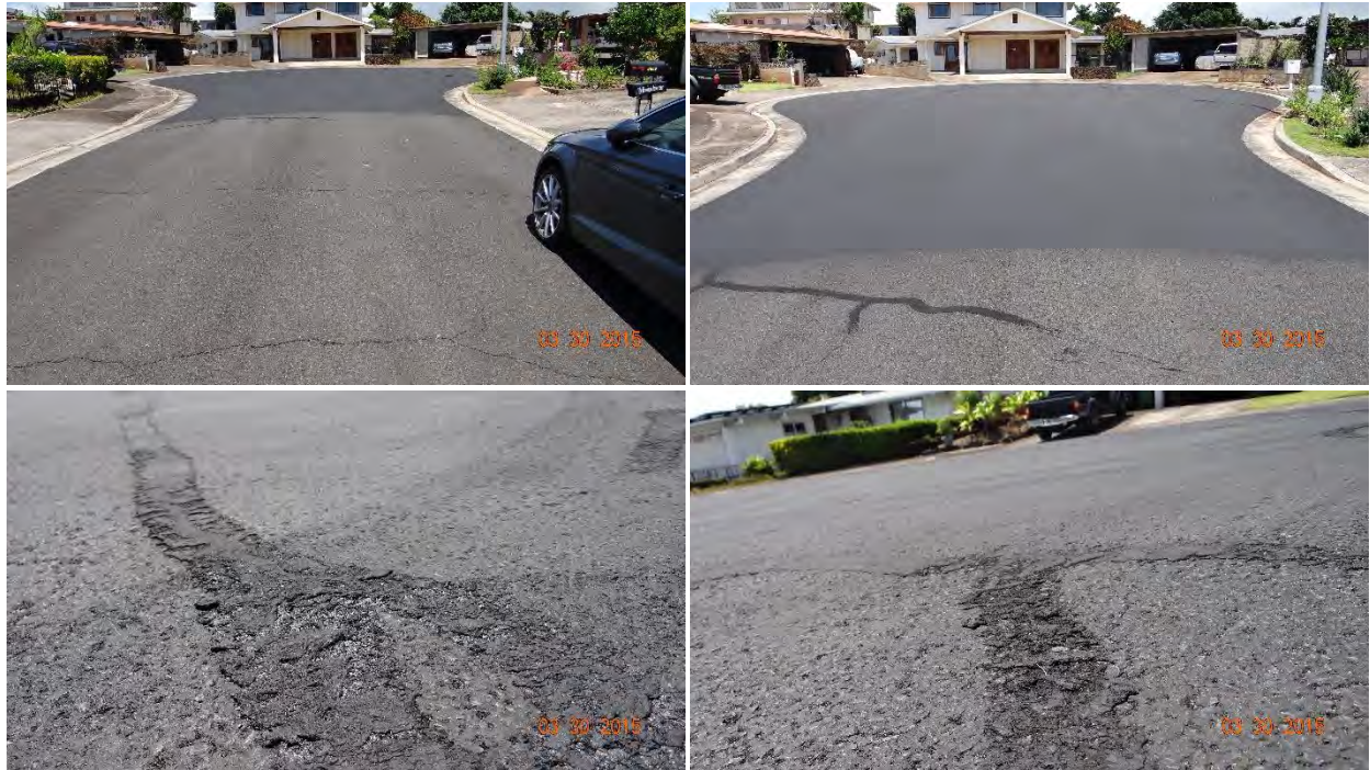
Figure C-126 Condition of the section on Hooheno Street, treated with Resurfacer by Brewer Cote (work performed by Oahu Seal Coating and Paving), on 3/30/2015.
