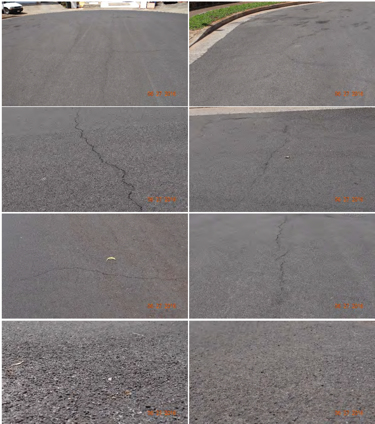
Figure C-149 Condition of the section on Hiana Place, treated with Slurry Seal by Alakona Corp., on 6/27/2016.
