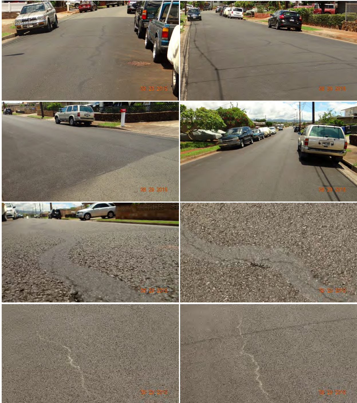
Figure C-52 Condition of Kaweloka Street section 1, treated with Plasti-Pave, on 08/29/2015.
