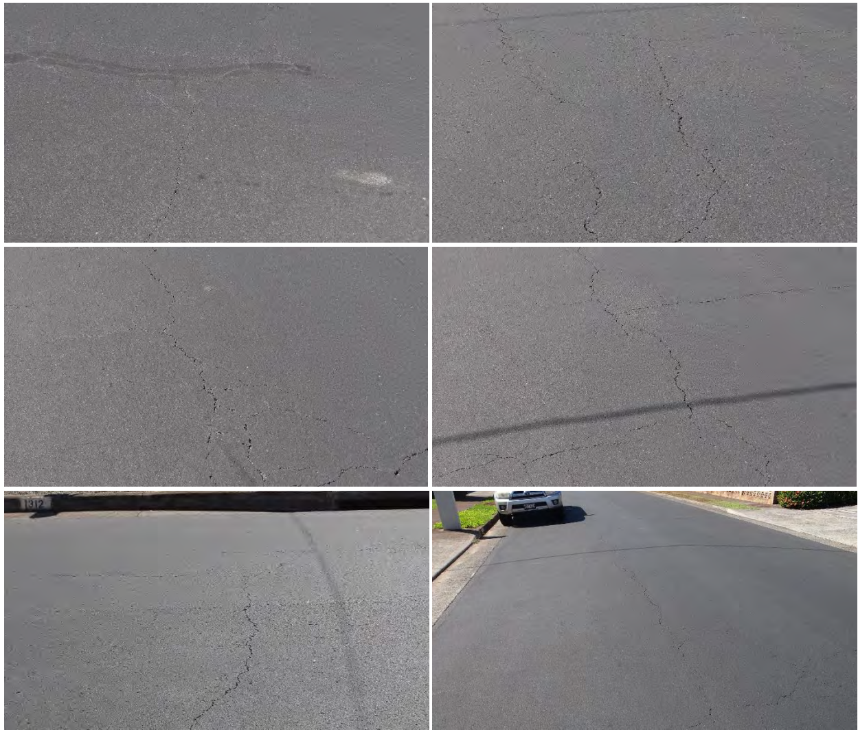
Figure C-74 Condition of Kaweloka Street section 3, treated with MasterSeal™ RTU, on 1/26/2018.
