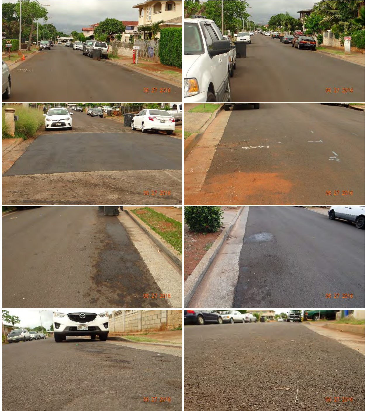
Figure C-141 Condition of the section on Hulahe Street, treated with Slurry Seal by Alakona Corp., on 6/27/2016.
