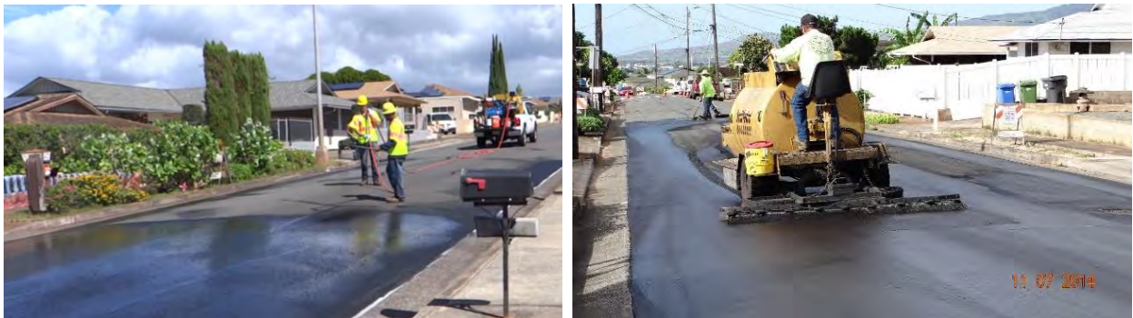
Figure 3-25 Application of seal coats: Manual spraying (left) and Spreader (right).
