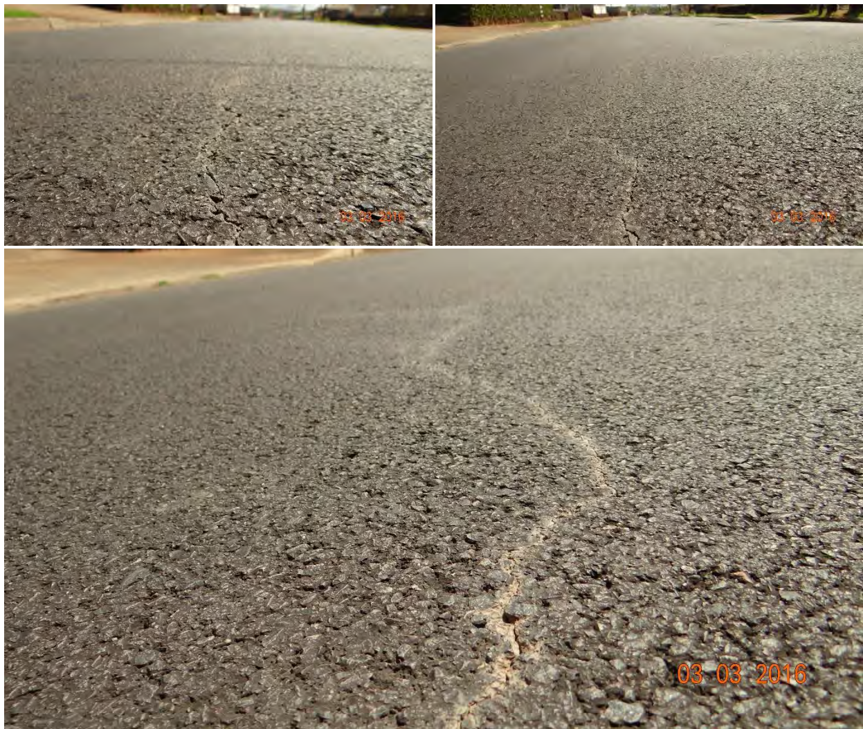
Figure C-53 Condition of Kaweloka Street section 1, treated with Plasti-Pave, on 03/3/2016.
