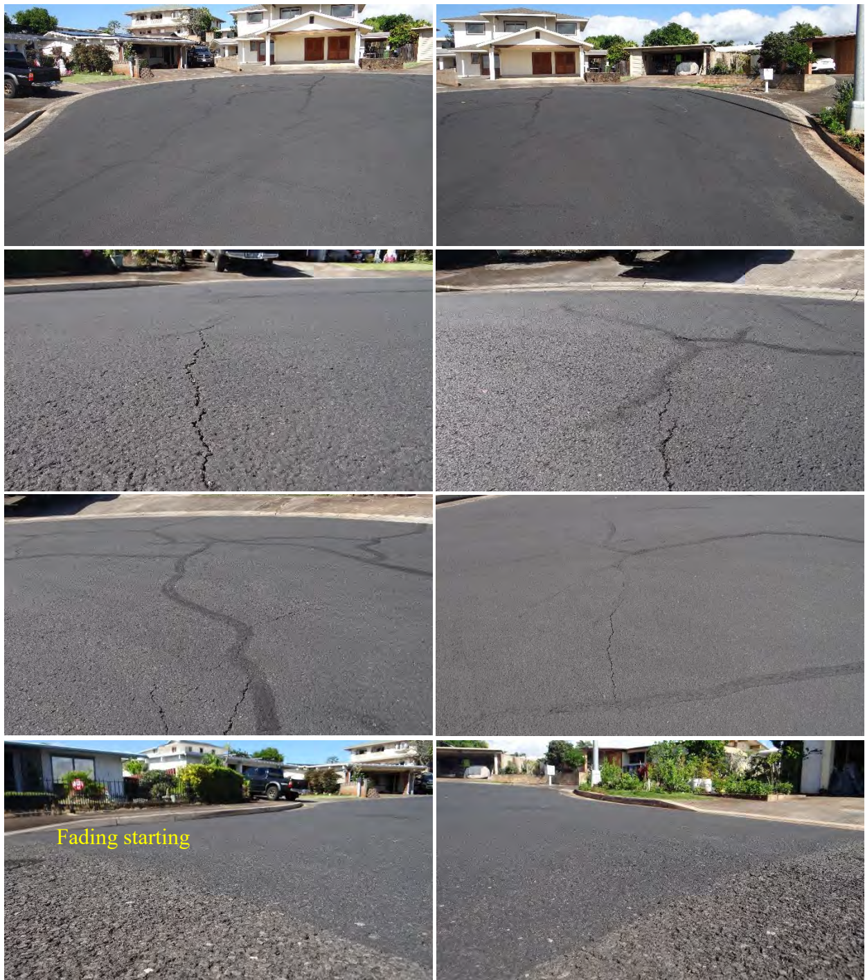
Figure C-129 Condition of the section on Hooheno Street, treated with Resurfacer by Brewer Cote (work performed by Oahu Seal Coating and Paving), on 12/14/2016.
