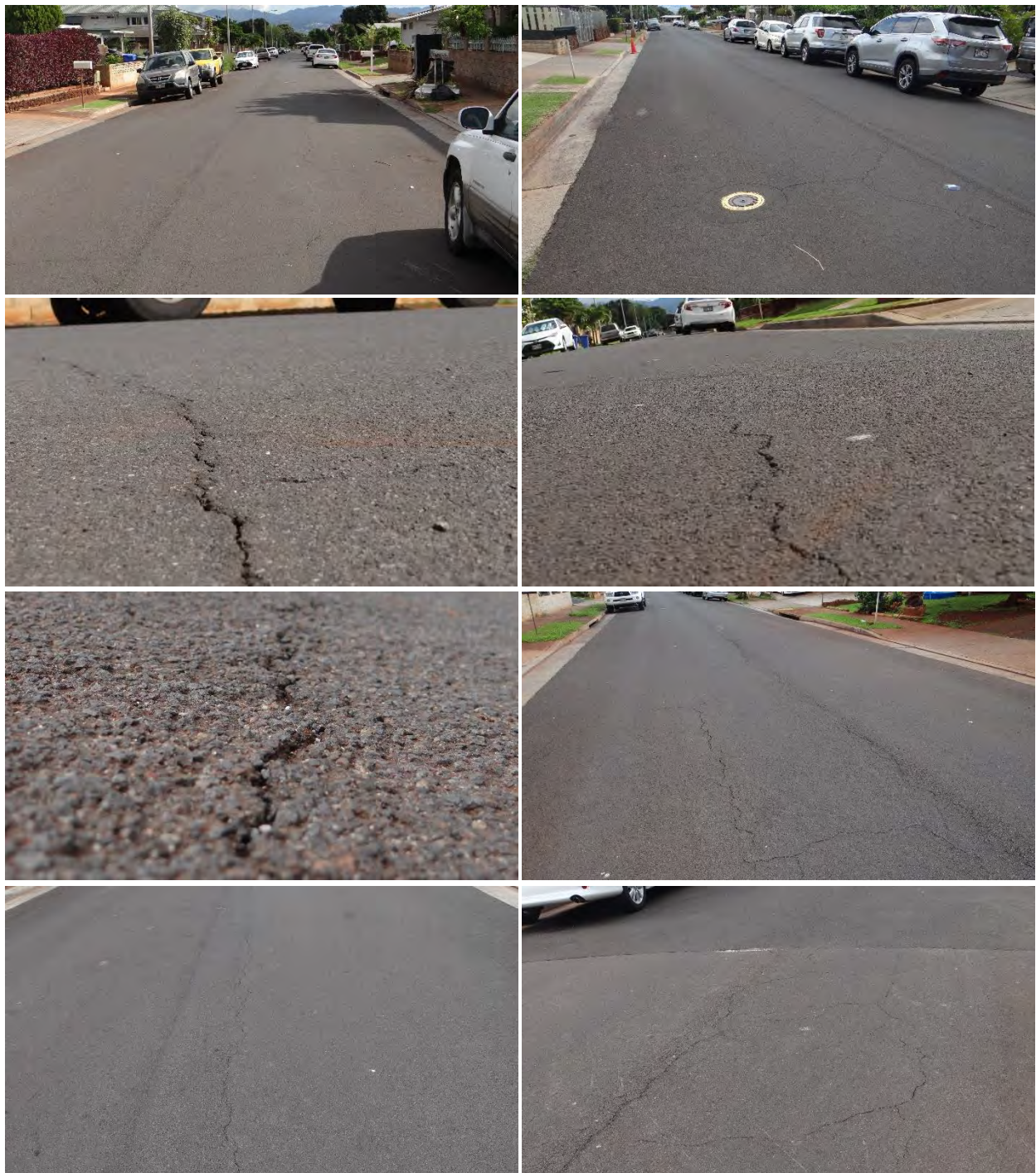
Figure C-144 Condition of the section on Hulahe Street, treated with Slurry Seal by Alakona Corp., on 2/7/2018.
