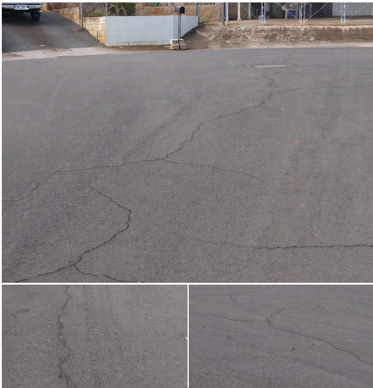
Figure C-157 Condition of the section on Hapapa Place, treated with Slurry Seal by Alakona Corp., on 12/14/2016.
