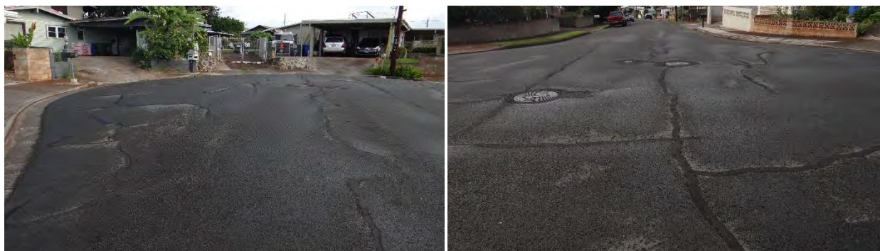
Figure C-98 Condition of the control section on Kaumoli Street on 12/13/2016.
