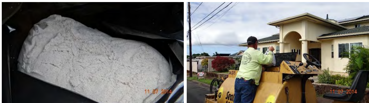
Figure 3-20 Sand used in seal coat and mixing of sand and emulsion.
