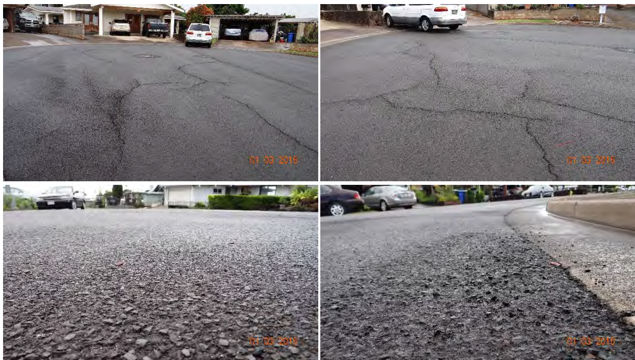
Figure C-125 Condition of the section on Hooheno Street, before treatment with Resurfacer by Brewer Cote (work performed by Oahu Seal Coating and Paving), on 1/3/2015.
