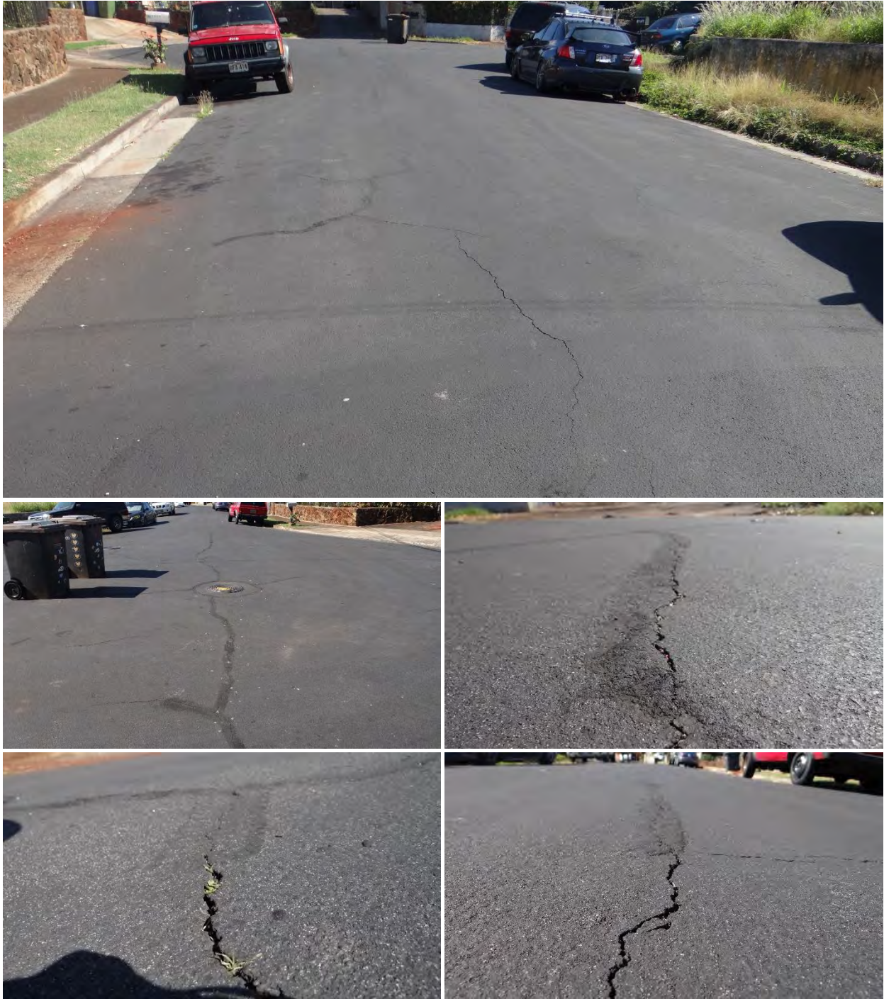
Figure C-109 Condition of the section on Kanihi Street, treated with Liquid Road, on 1/26/2018.
