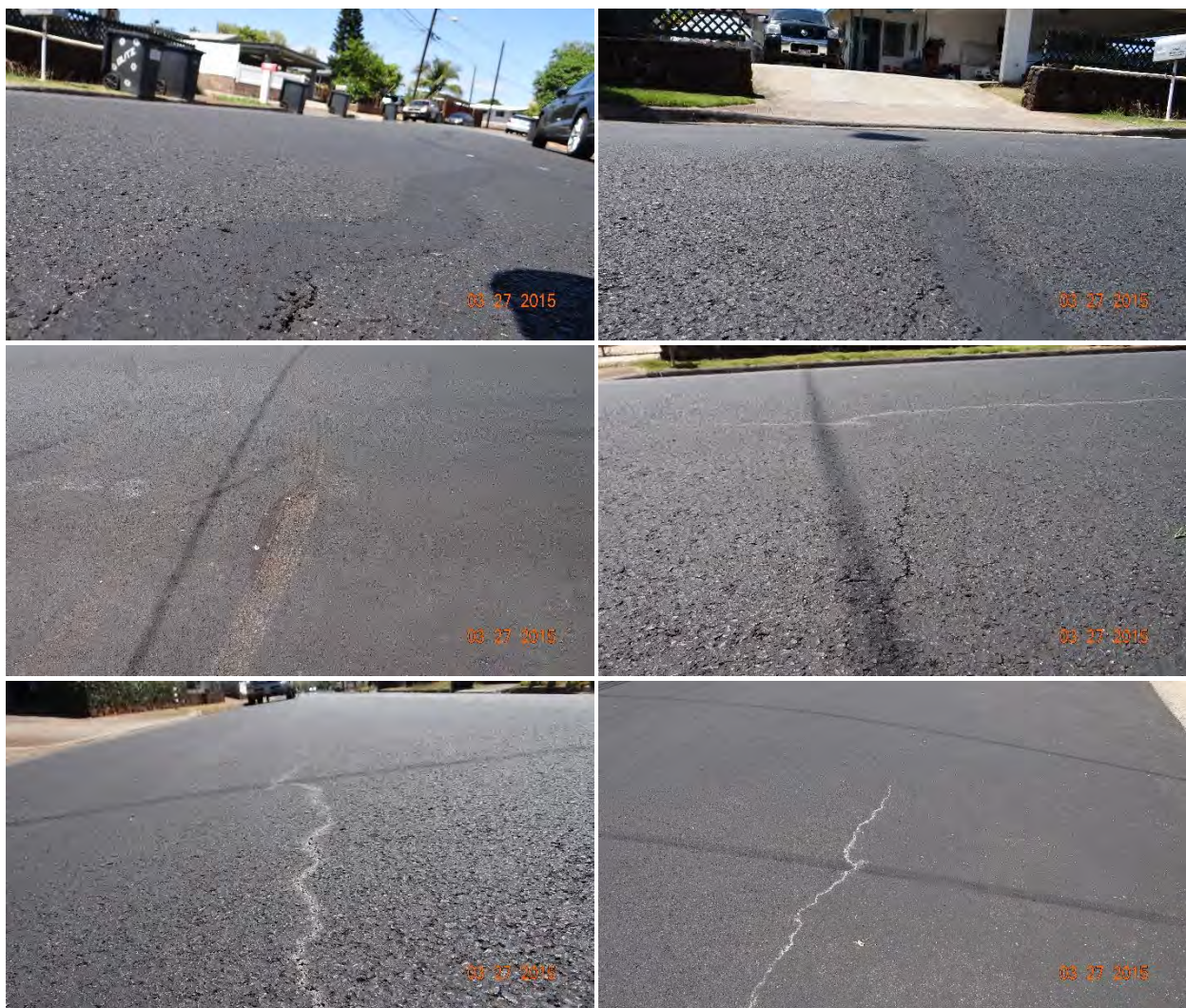
Figure C-51 Condition of Kaweloka Street section 1, treated with Plasti-Pave, on 03/27/2015.
