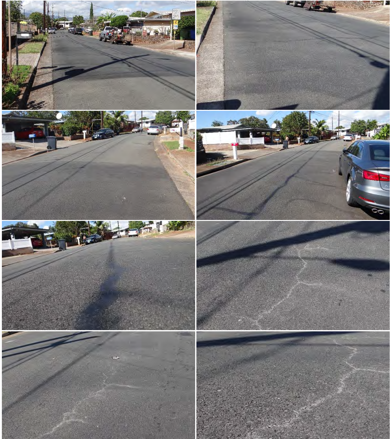
Figure C-56 Condition of Kaweloka Street section 1, treated with Plasti-Pave, on 1/26/2018.
