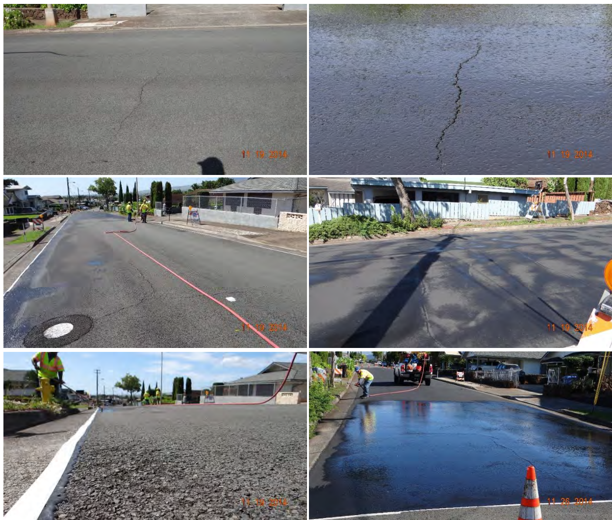
Figure C-87 Condition of section 5 on Kaweloka Street, treated with CarbonSeal-HT, on 11/19/2014 and 11/26/2014.
