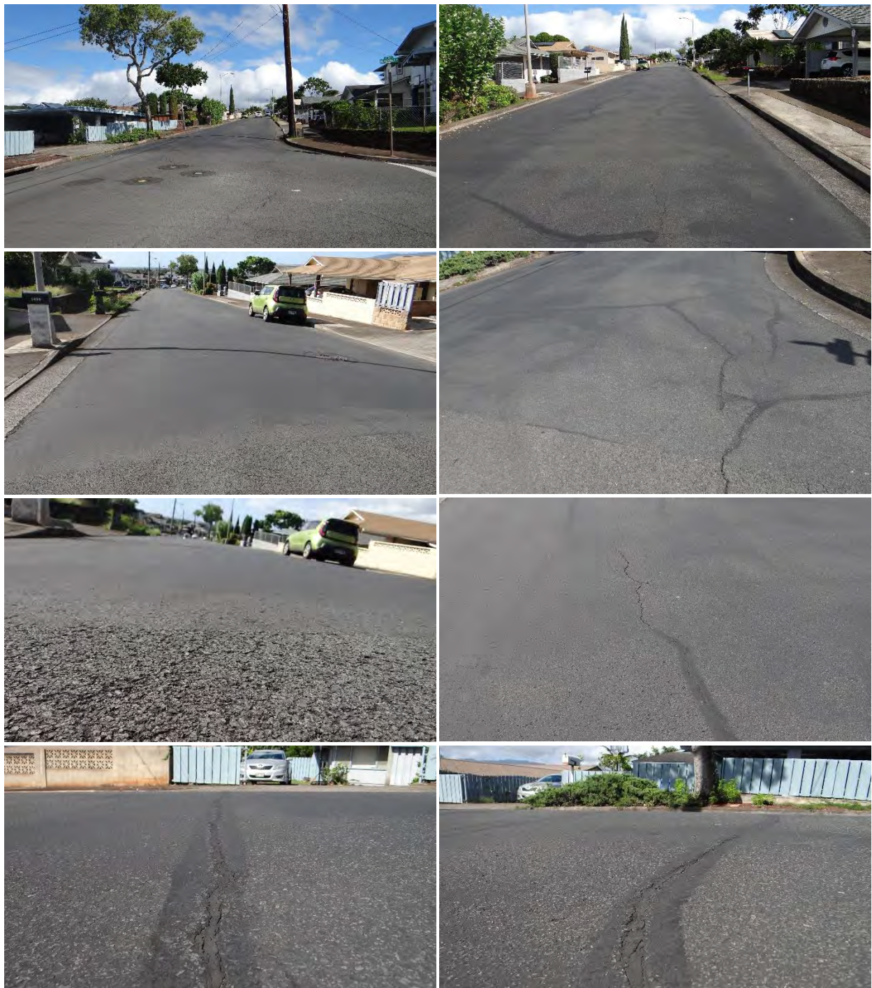
Figure C-90 Condition of section 5 on Kaweloka Street, treated with CarbonSeal-HF, on 6/24/2016.
