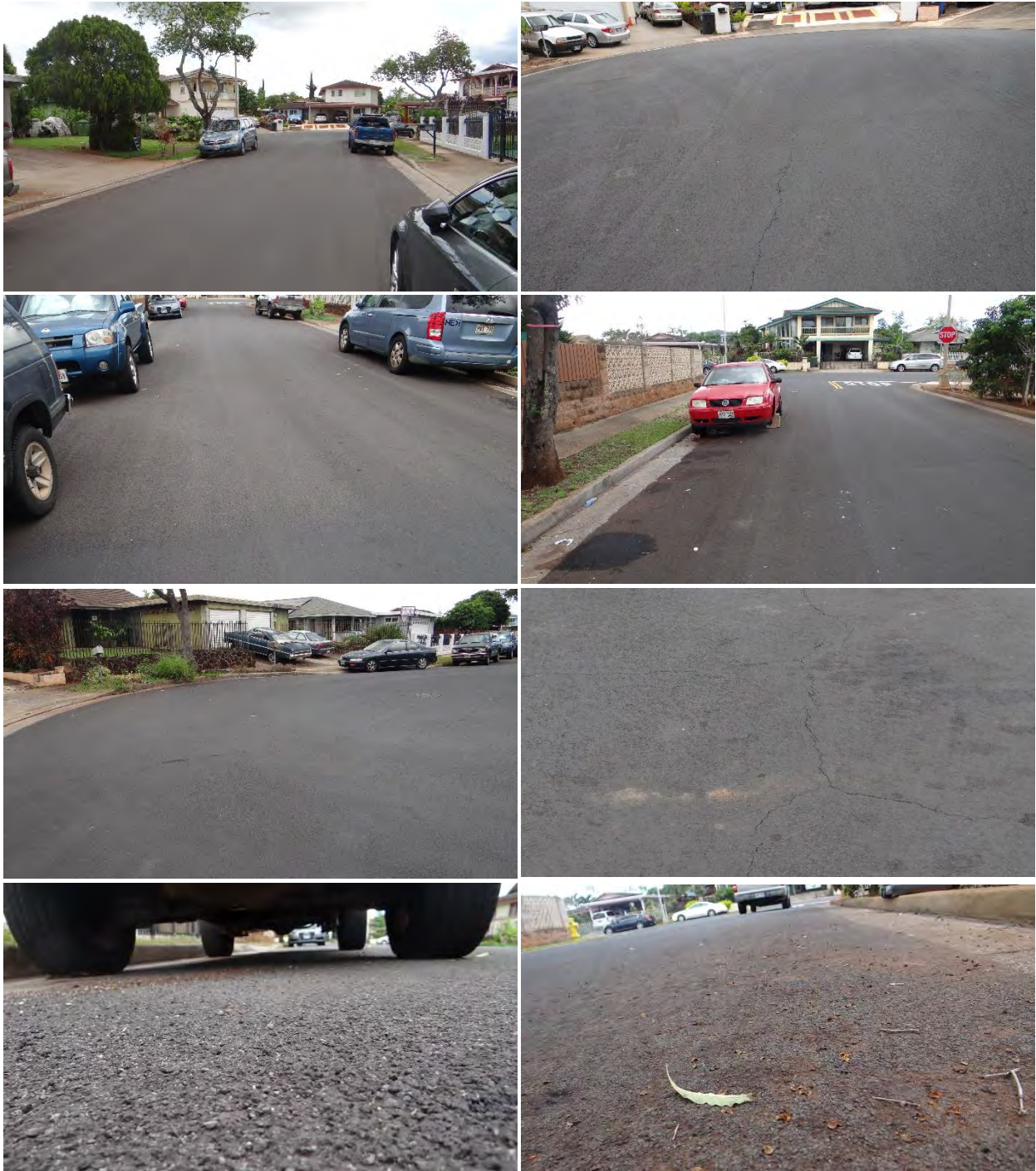
Figure C-151 Condition of the section on Hiana Place, treated with Slurry Seal by Alakona Corp., on 2/7/2018.
