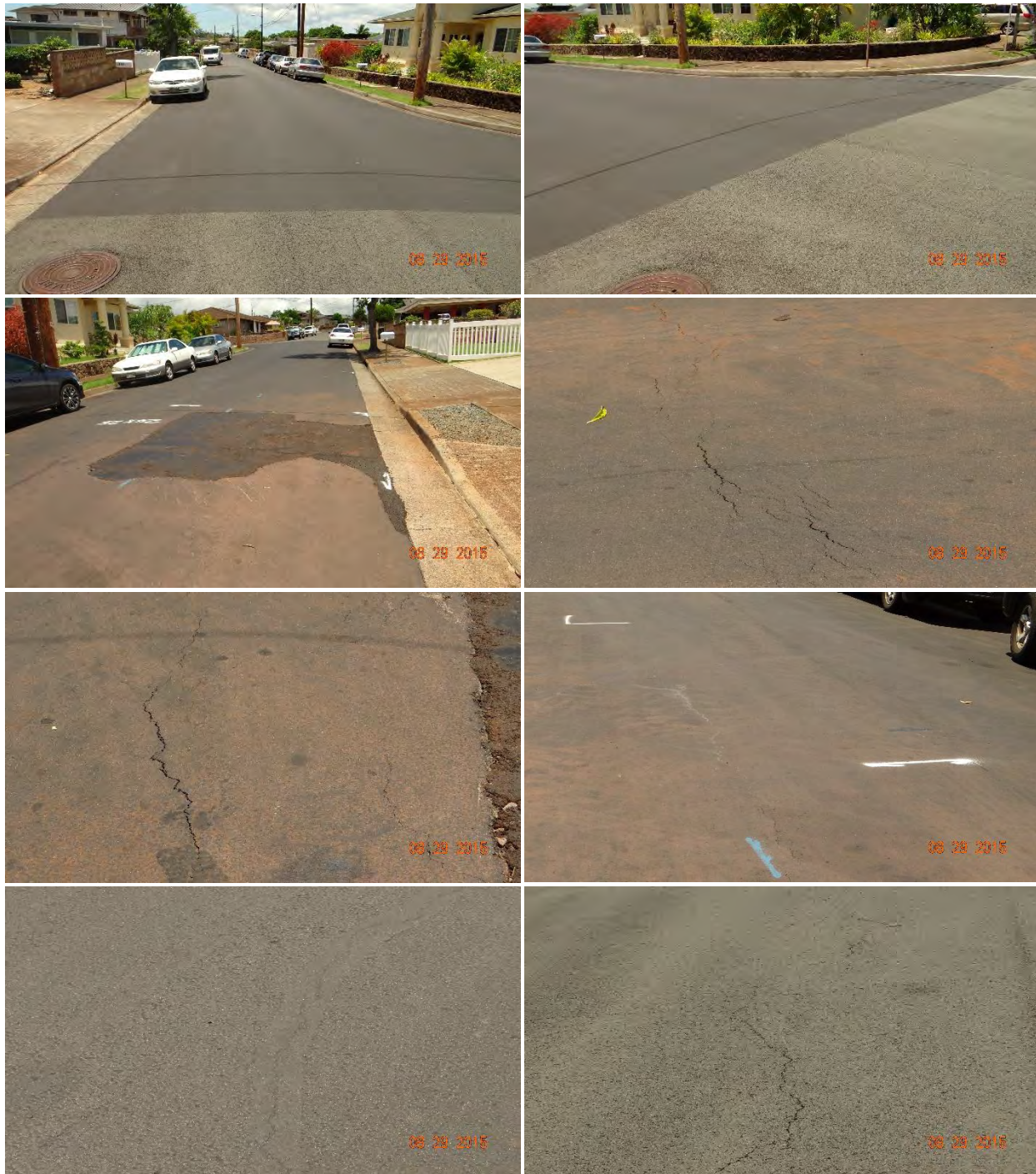
Figure C-70 Condition of Kaweloka Street section 3, treated with MasterSeal™ RTU, on 8/29/2015.
