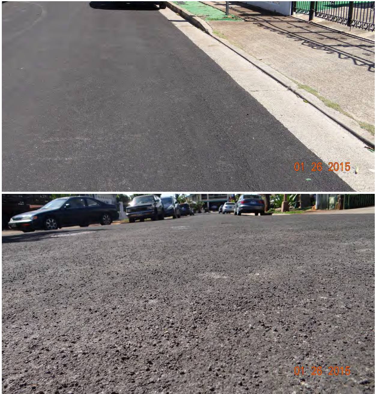
Figure C-146 Condition of the section on Hiana Place, treated with Slurry Seal by Alakona Corp., on 1/26/2015.
