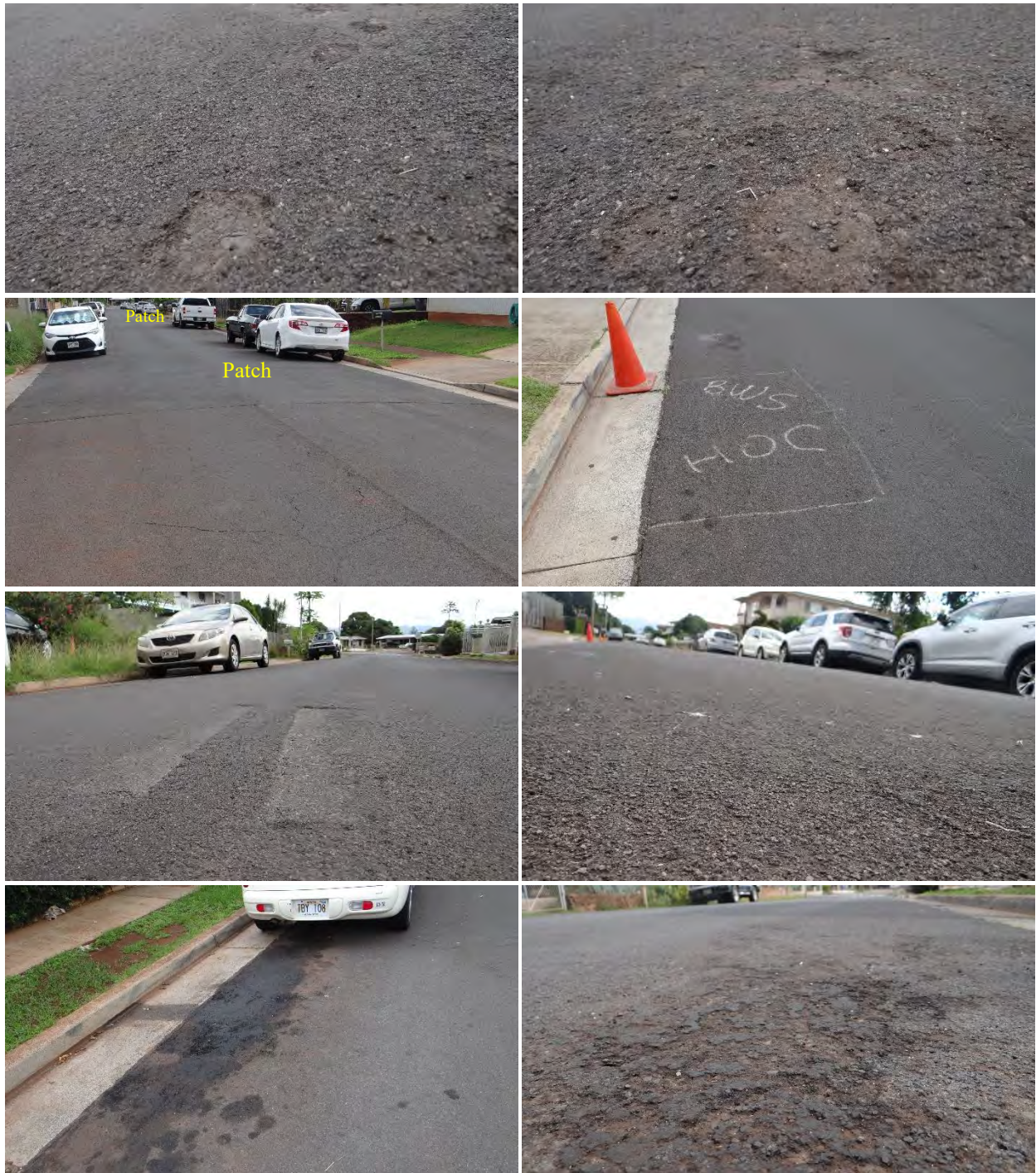
Figure C-145 Condition of the section on Hulahe Street, treated with Slurry Seal by Alakona Corp., on 2/7/2018.
