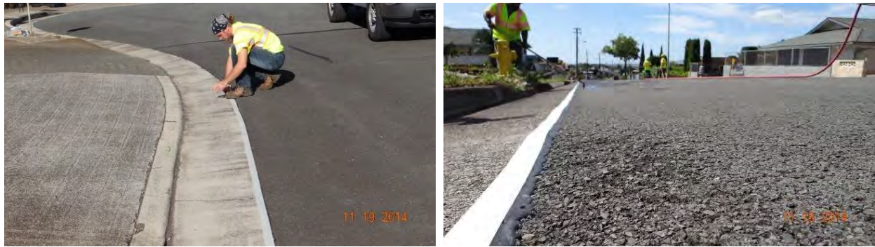
Figure 3-18 Use of tape to avoid spreading of the emulsion into the gutter.
