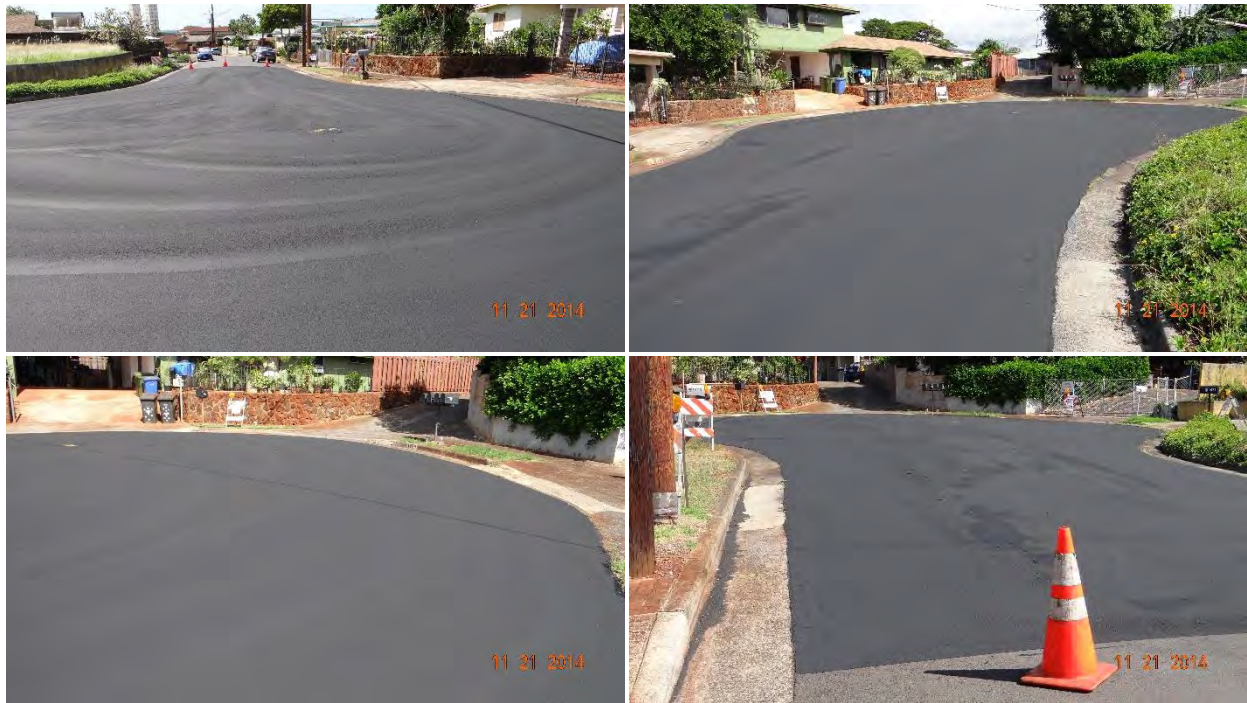
Figure C-104 Condition of the section on Kanihi Street, treated with Liquid Road, on 11/21/2014.
