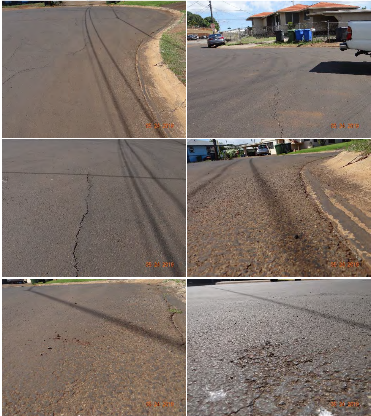
Figure C-103 Condition of the section on Hoolawa Place, treated with Plasti-Pave, on 5/24/2019.
