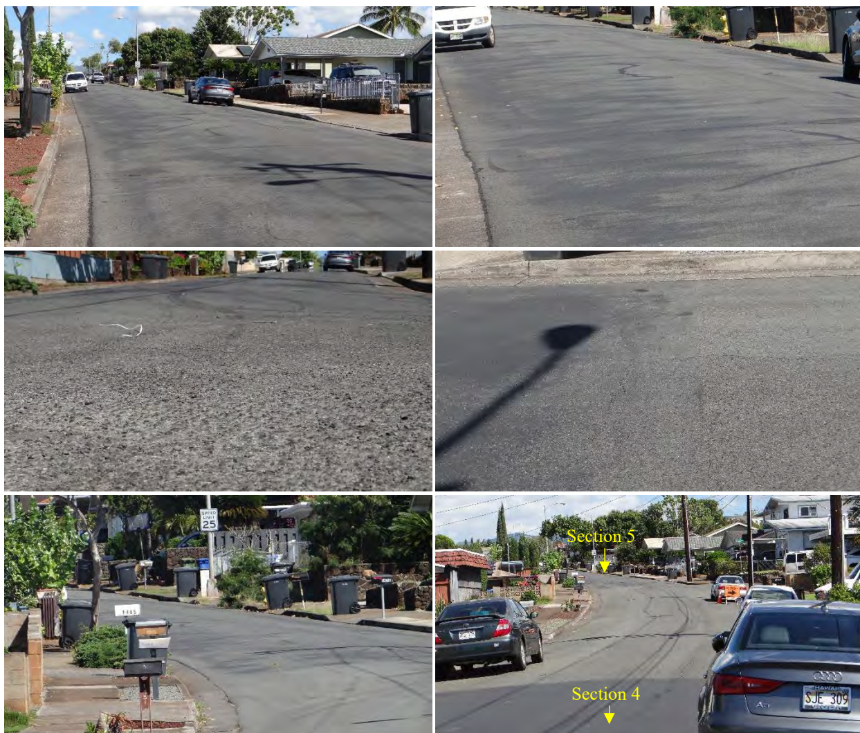
Figure C-91 Condition of section 5 on Kaweloka Street, treated with CarbonSeal-HF, on 1/26/2018.
