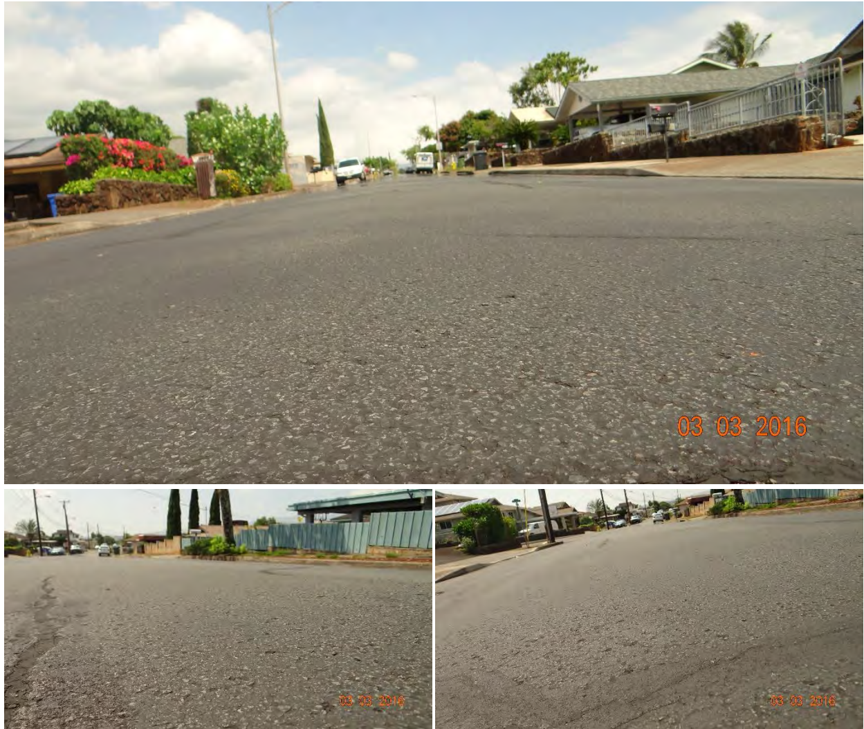
Figure C-89 Condition of section 5 on Kaweloka Street, treated with CarbonSeal-HF, on 3/3/2016.
