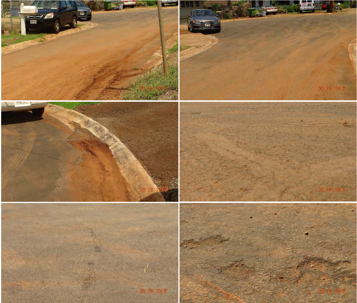
Figure C-100 Condition of the section on Hoolawa Place, treated with Plasti-Pave, on 8/29/2015.
