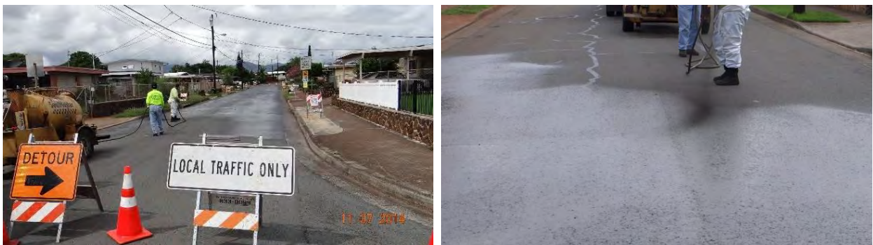
Figure 3-26 Pavement rejuvenator application.
