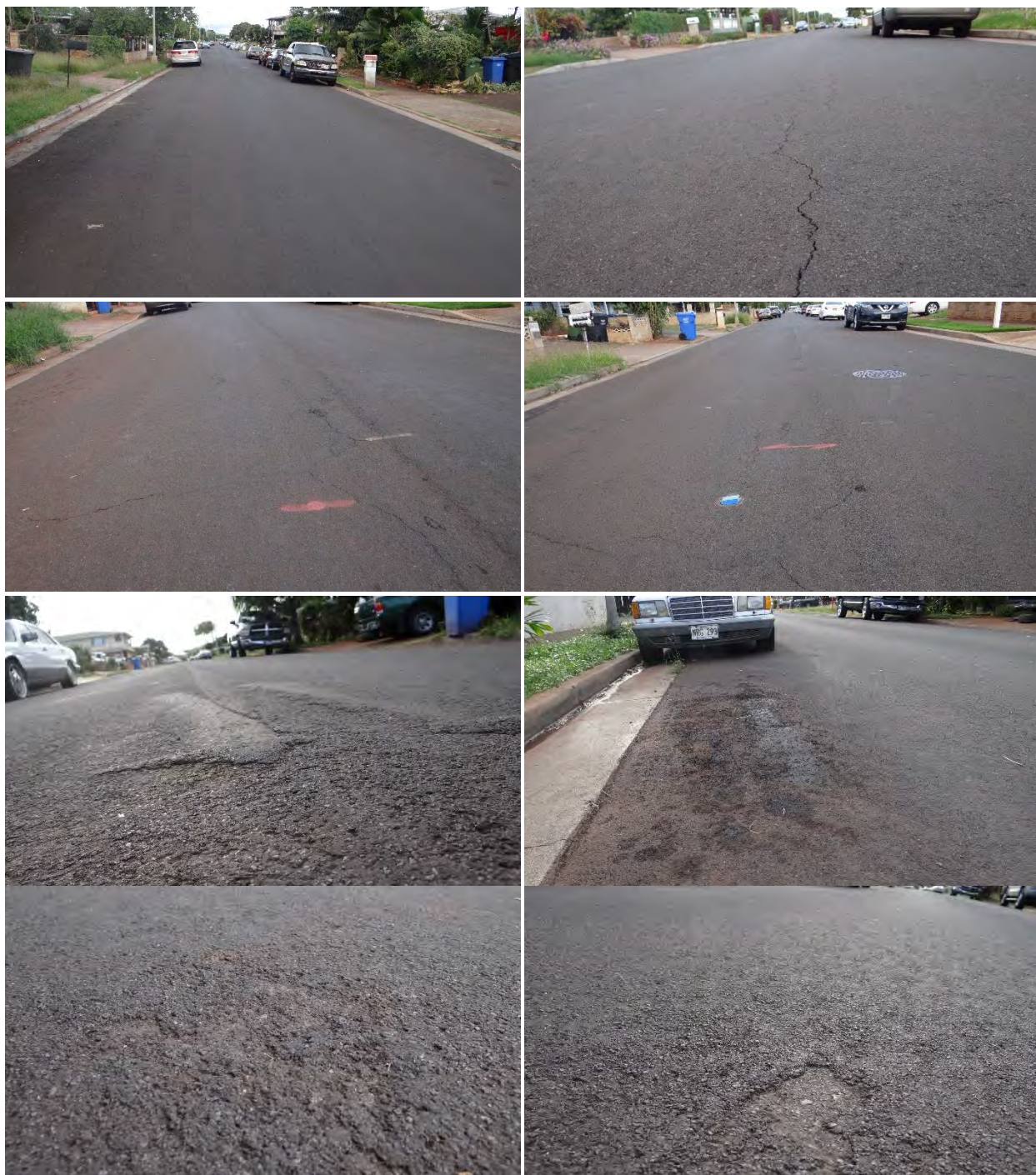
Figure C-143 Condition of the section on Hulahe Street, treated with Slurry Seal by Alakona Corp., on 12/14/2016.
