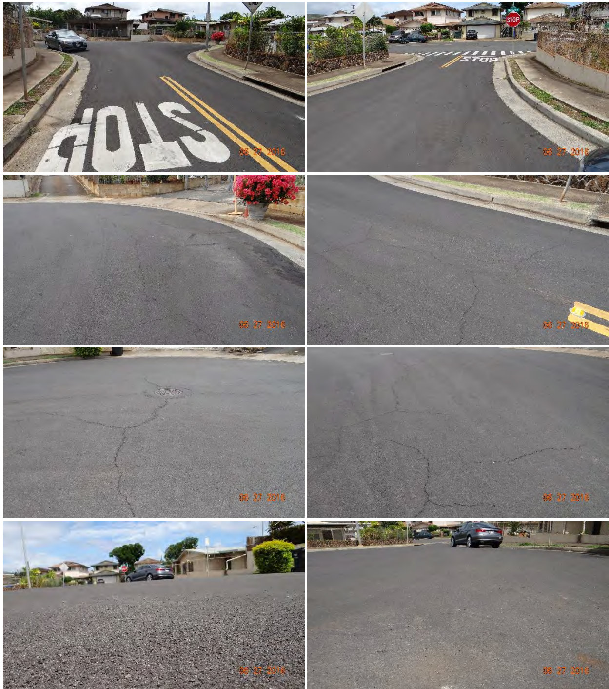
Figure C-156 Condition of the section on Hapapa Place, treated with Slurry Seal by Alakona Corp., on 6/27/2016.
