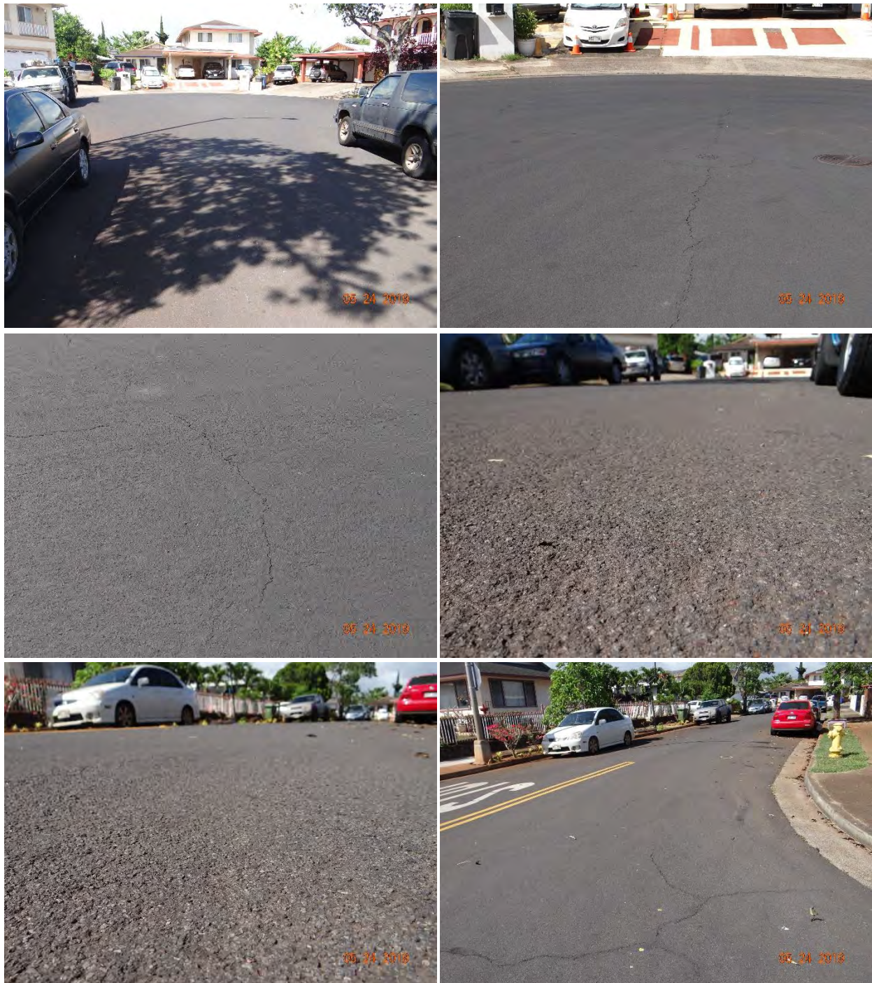
Figure C-152 Condition of the section on Hiana Place, treated with Slurry Seal by Alakona Corp., on 5/24/2019.
