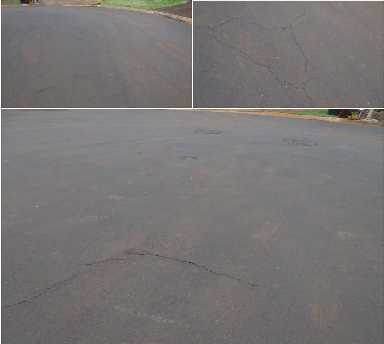
Figure C-102 Condition of the section on Hoolawa Place, treated with Plasti-Pave, on 2/7/2018.
