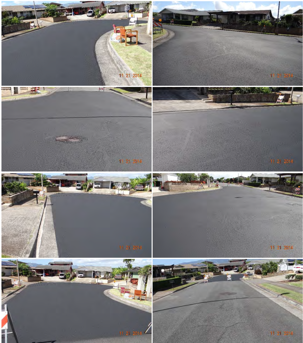
Figure C-111 Condition of the section on Kalauipo Place, treated with MasterSeal™ Ready to Use, on 11/21/2014.
