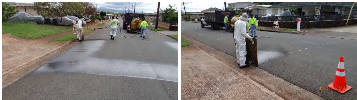
Figure 3-19 Use of a board to avoid spreading of the emulsion into the gutter.
