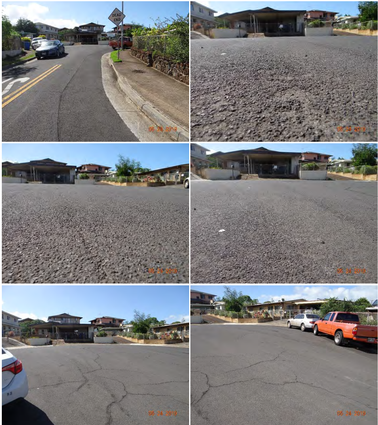
Figure C-159 Condition of the section on Hapapa Place, treated with Slurry Seal by Alakona Corp., on 5/24/2019.
