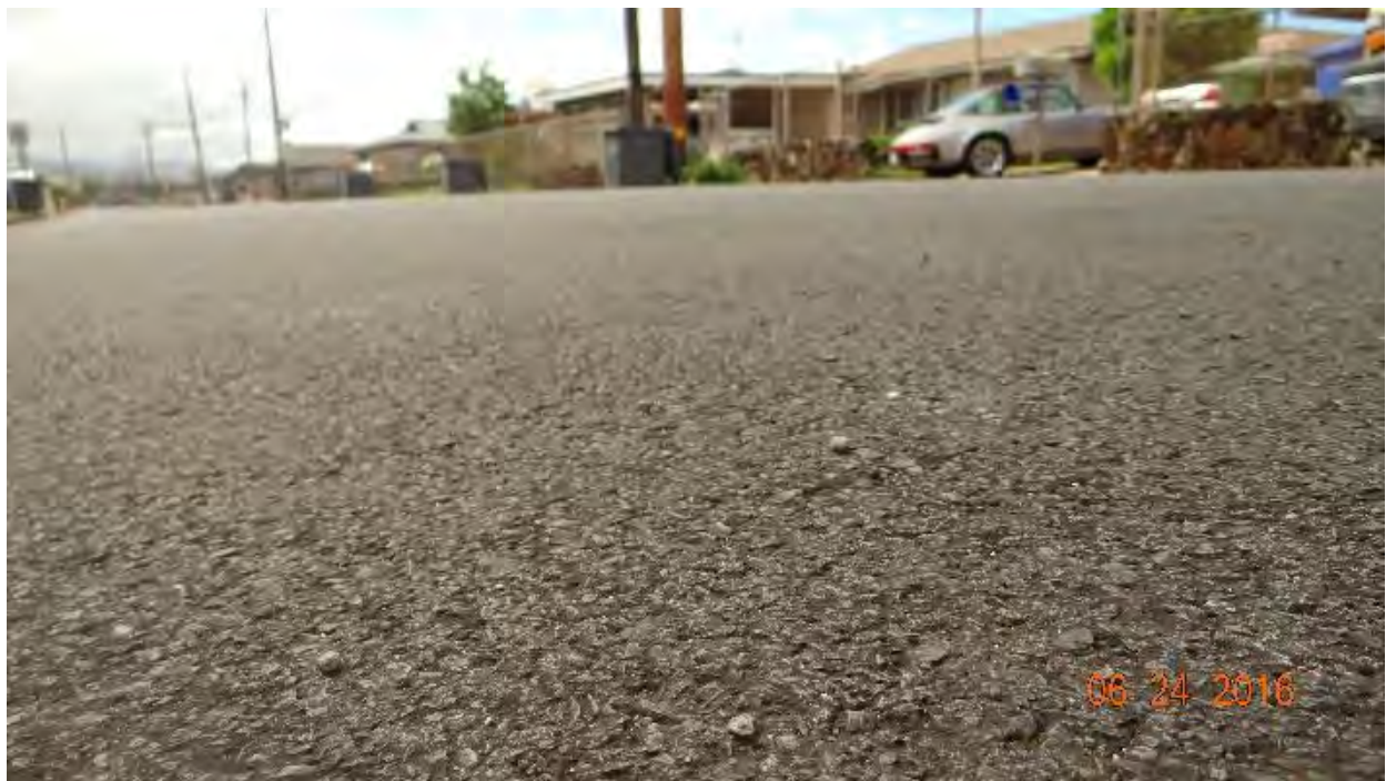
Figure C-54 Condition of Kaweloka Street section 1, treated with Plasti-Pave, on 06/24/2016.
