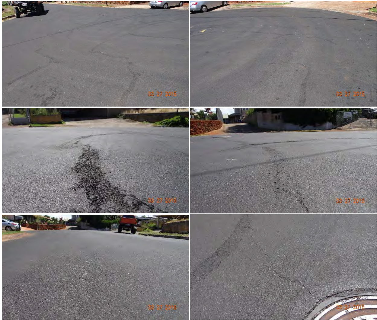
Figure C-105 Condition of the section on Kanihi Street, treated with Liquid Road, on 3/27/2015.
