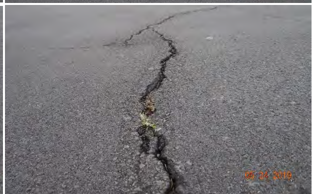
Figure C-110 Condition of the section on Kanihi Street, treated with Liquid Road, on 5/24/2019.
