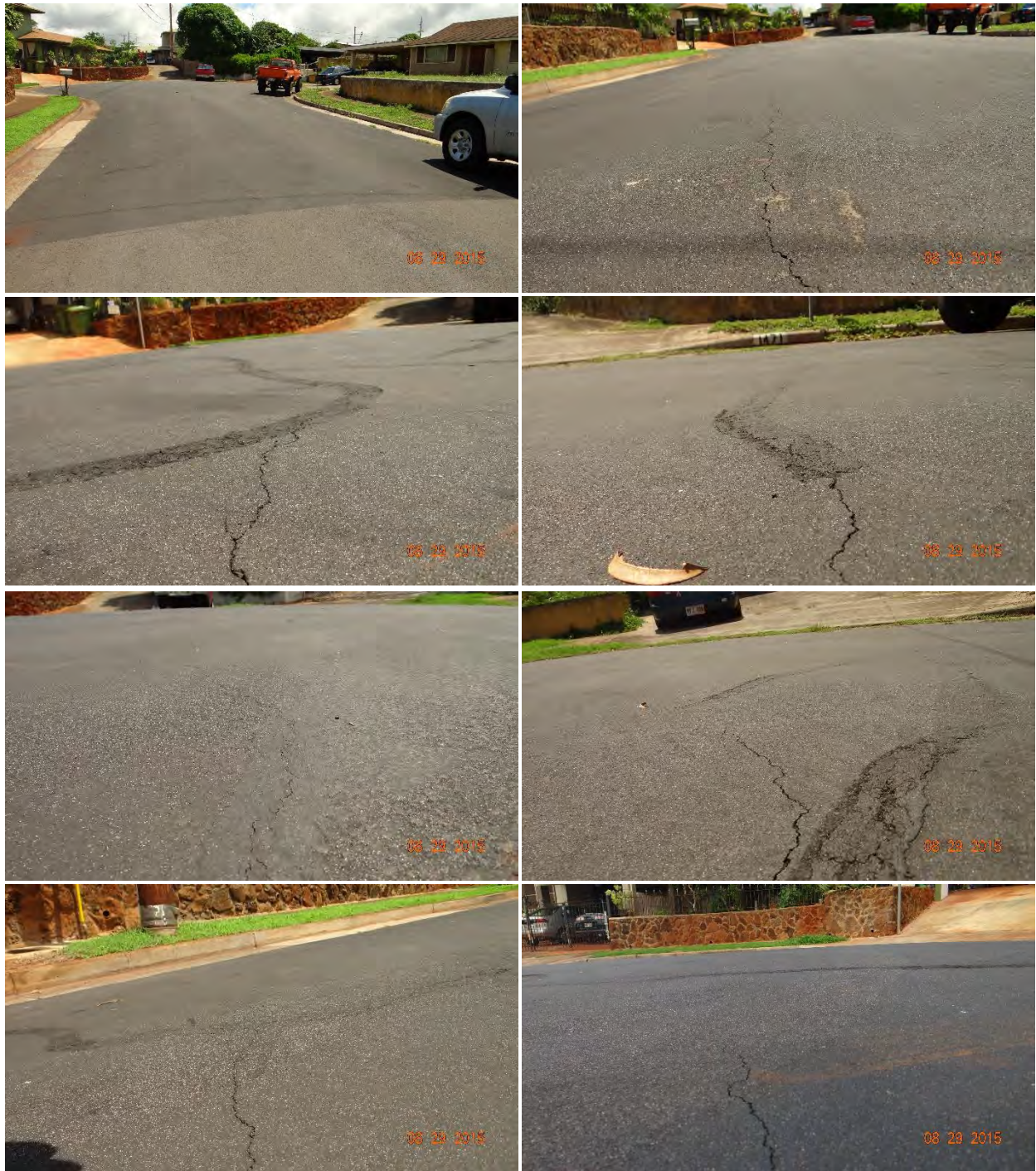
Figure C-106 Condition of the section on Kanihi Street, treated with Liquid Road, on 8/29/2015.
