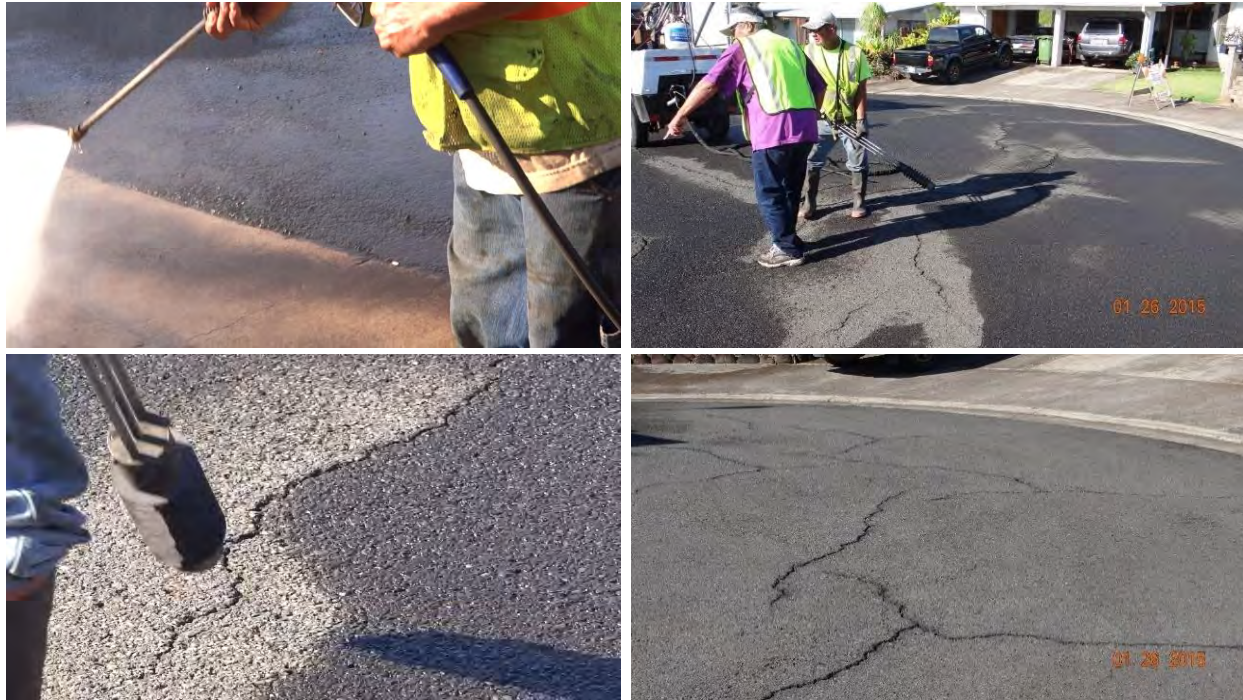
Figure 3-22 Use of power washing to clean the pavement surface.
