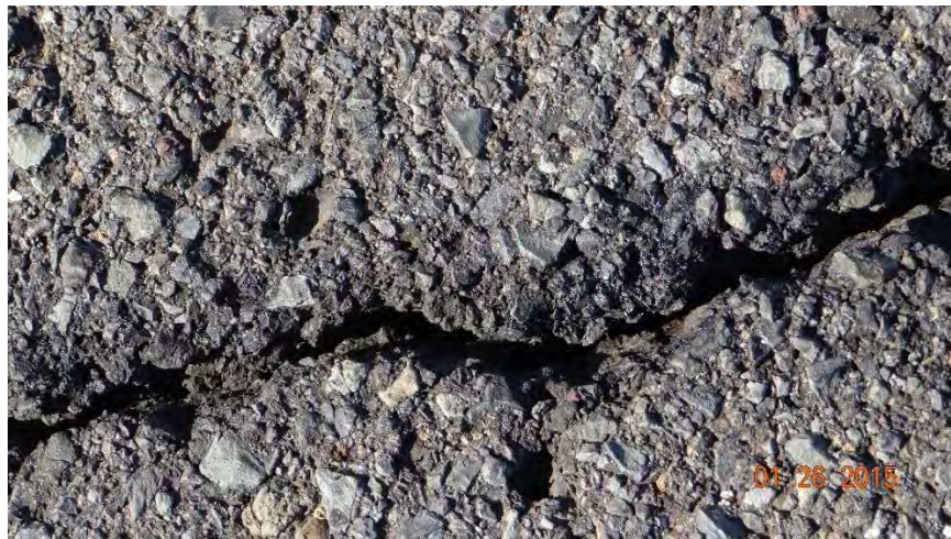
Figure 3-23 Very clean crack obtained by power washing.
