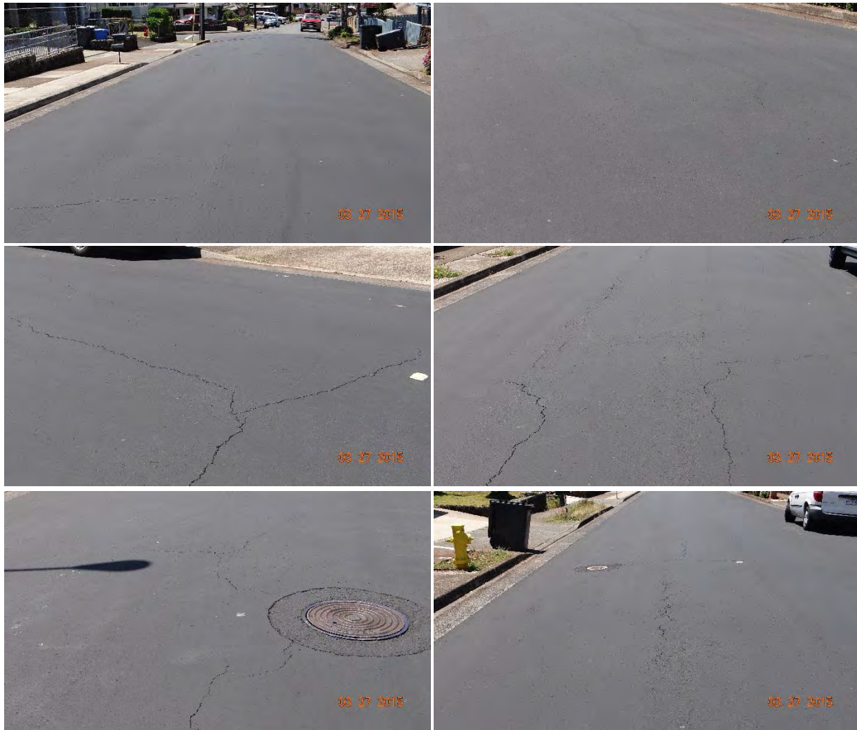
Figure C-88 Condition of section 5 on Kaweloka Street, treated with CarbonSeal-HF, on 3/27/2015.
