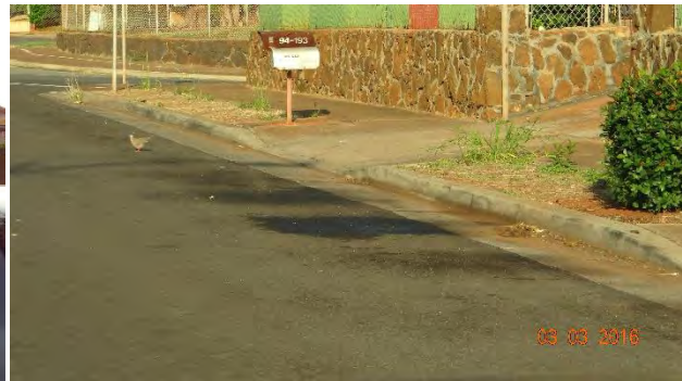
Figure C-140 Condition of the section on Hulahe Street, treated with Slurry Seal by Alakona Corp., on 3/3/2016.
