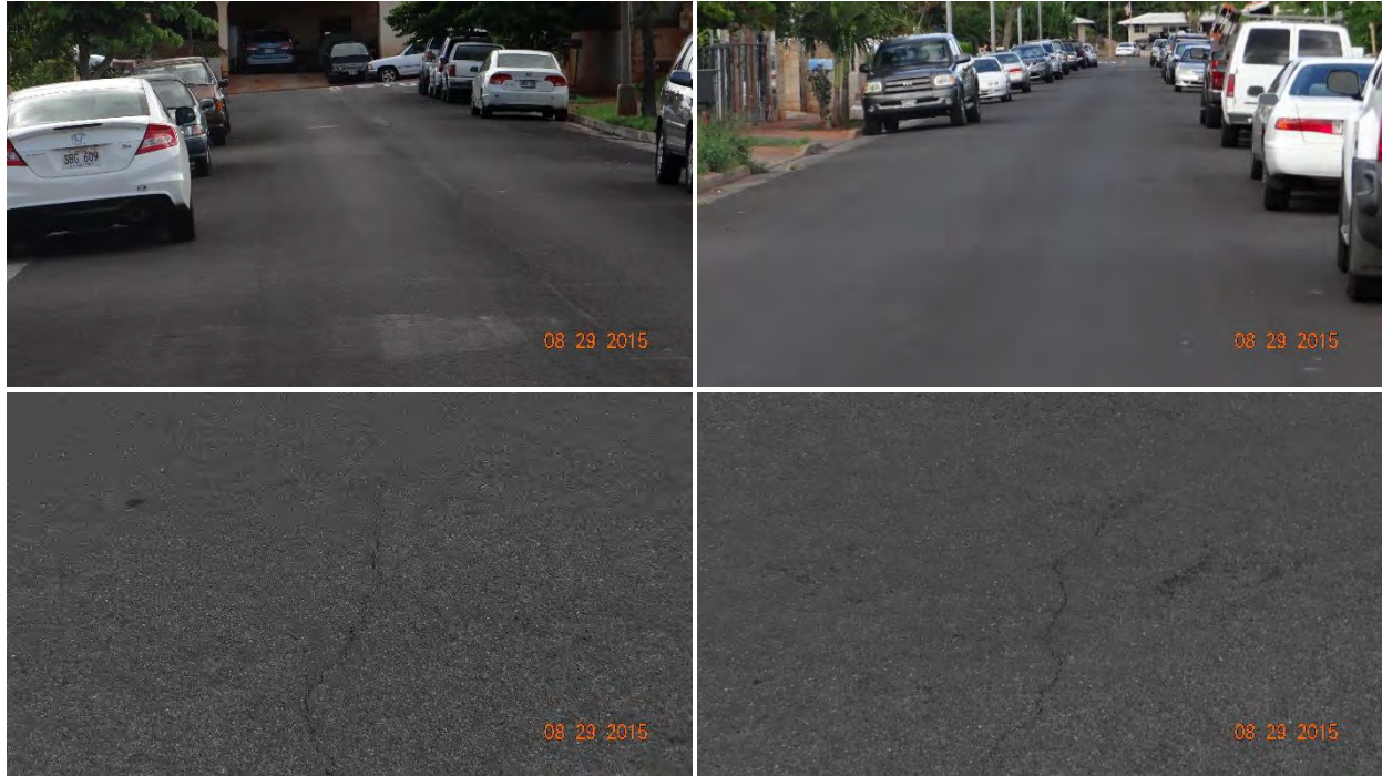
Figure C-139 Condition of the section on Hulahe Street, treated with Slurry Seal by Alakona Corp., on 8/29/2015.
