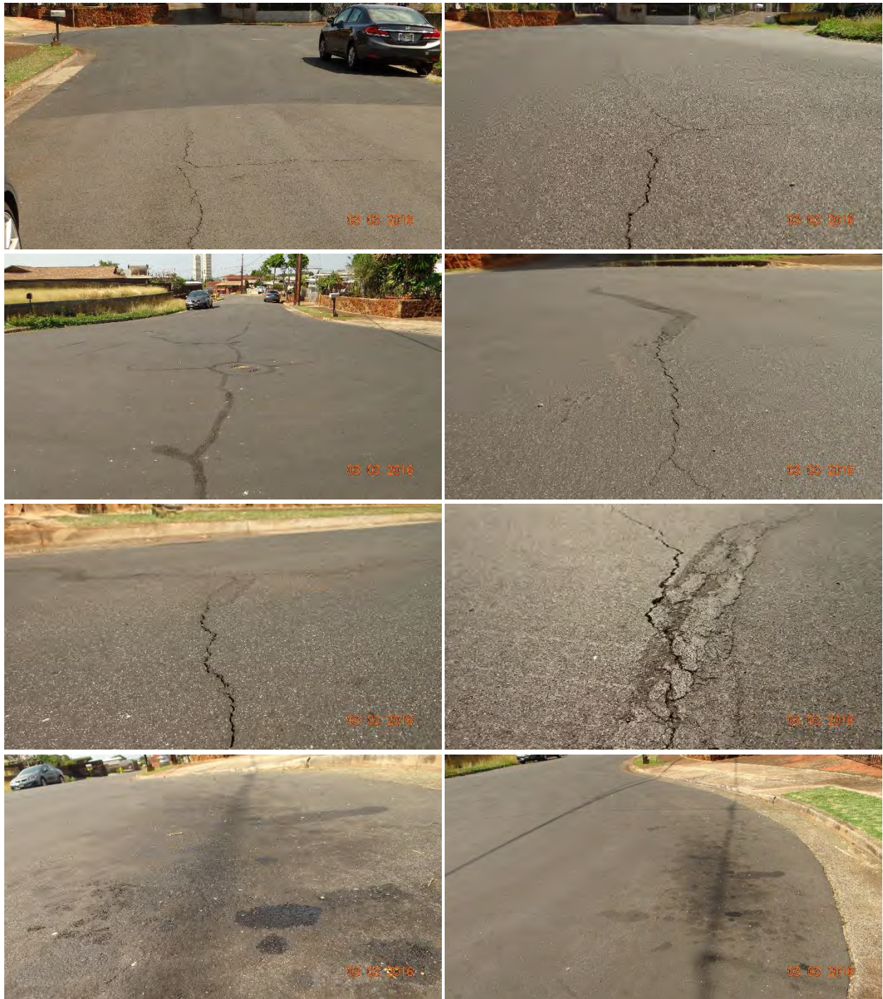
Figure C-107 Condition of the section on Kanihi Street, treated with Liquid Road, on 3/3/2016.
