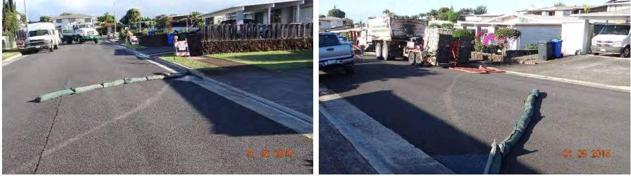
Figure 3-24 Environmental precautions for power washing.
