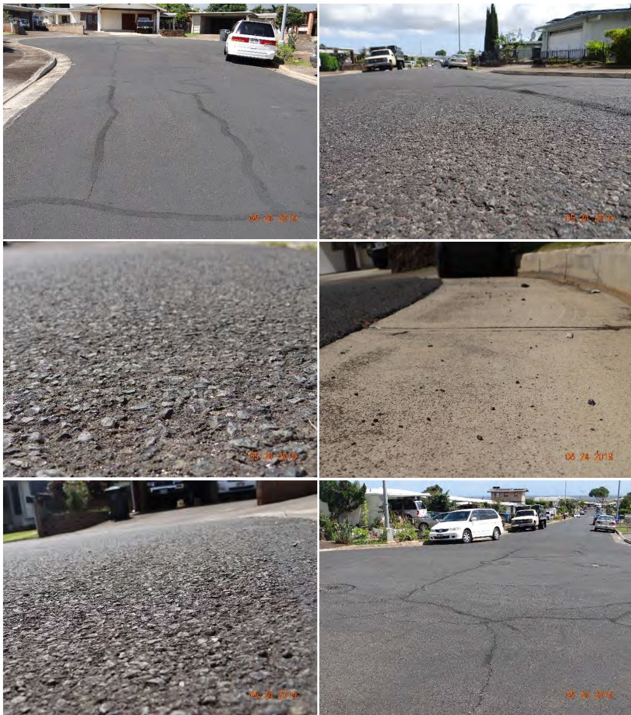
Figure C-131 Condition of the section on Hooheno Street, treated with Resurfacer by Brewer Cote (work performed by Oahu Seal Coating and Paving), on 5/24/2019.
