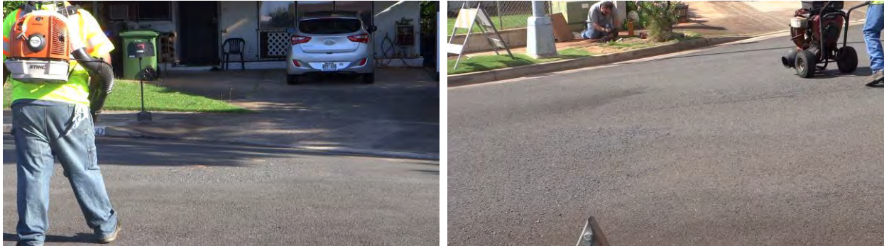
Figure 3-21 Use of blowers to clean the surface of loose aggregate and dust.
