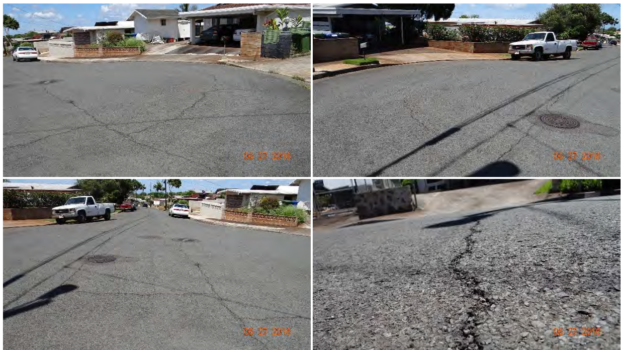
Figure C-97 Condition of the control section on Kaumoli Street on 6/27/2016.
