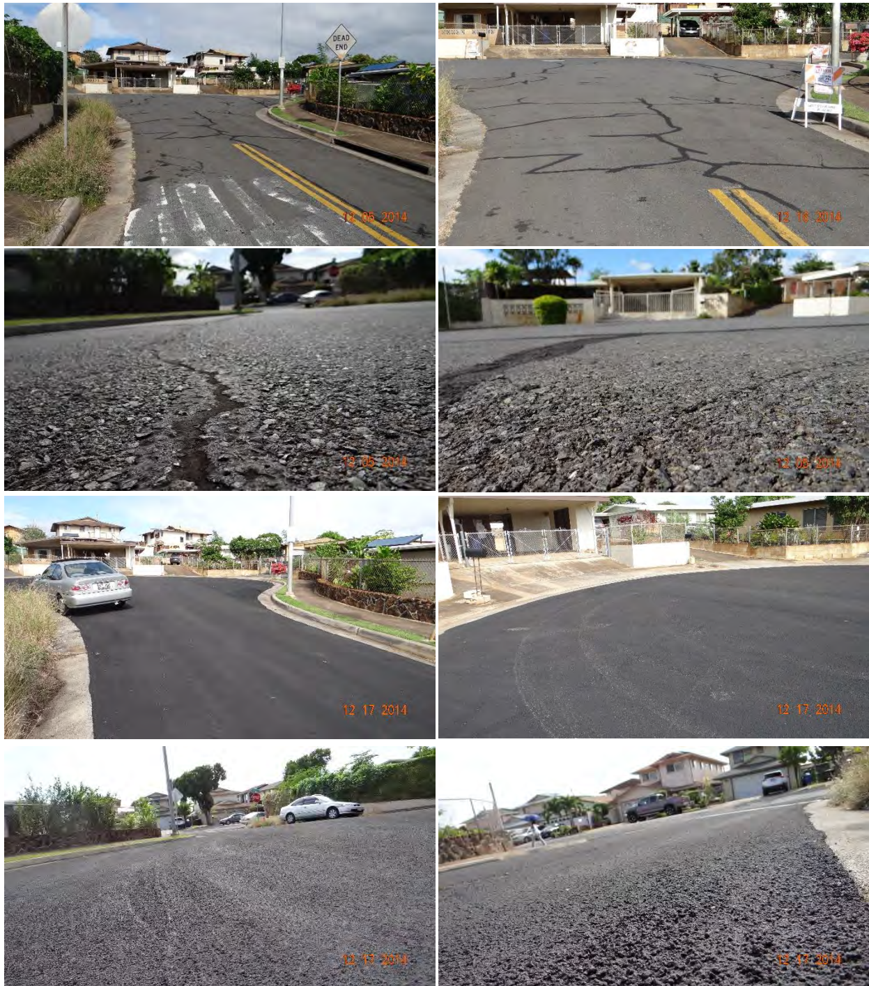
Figure C-153 Condition of the section on Hapapa Place, treated with Slurry Seal by Alakona Corp., on 12/5/2014 to 12/17/2014.
