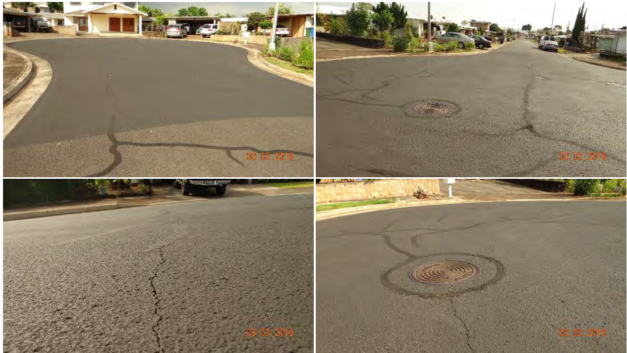
Figure C-128 Condition of the section on Hooheno Street, treated with Resurfacer by Brewer Cote (work performed by Oahu Seal Coating and Paving), on 3/3/2016.
