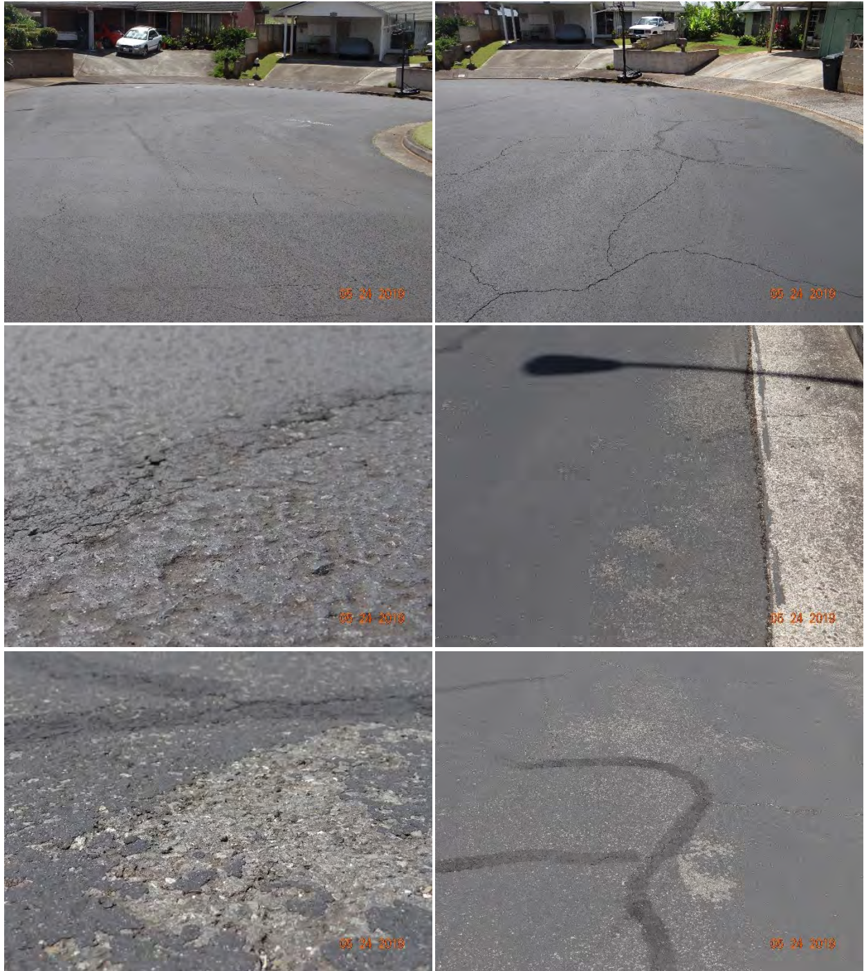
Figure C-117 Condition of the section on Kalauipo Place, treated with MasterSeal™ Ready to Use, on 5/24/2019.
