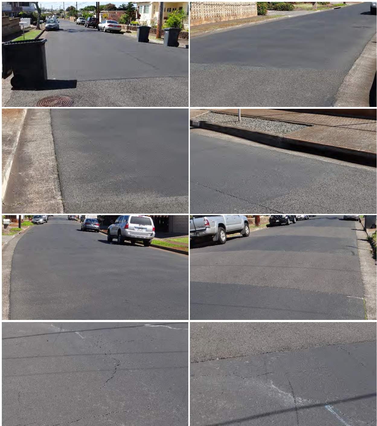
Figure C-73 Condition of Kaweloka Street section 3, treated with MasterSeal™ RTU, on 1/26/2018.
