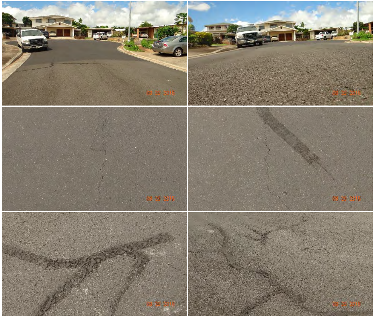
Figure C-127 Condition of the section on Hooheno Street, treated with Resurfacer by Brewer Cote (work performed by Oahu Seal Coating and Paving), on 8/29/2015.
