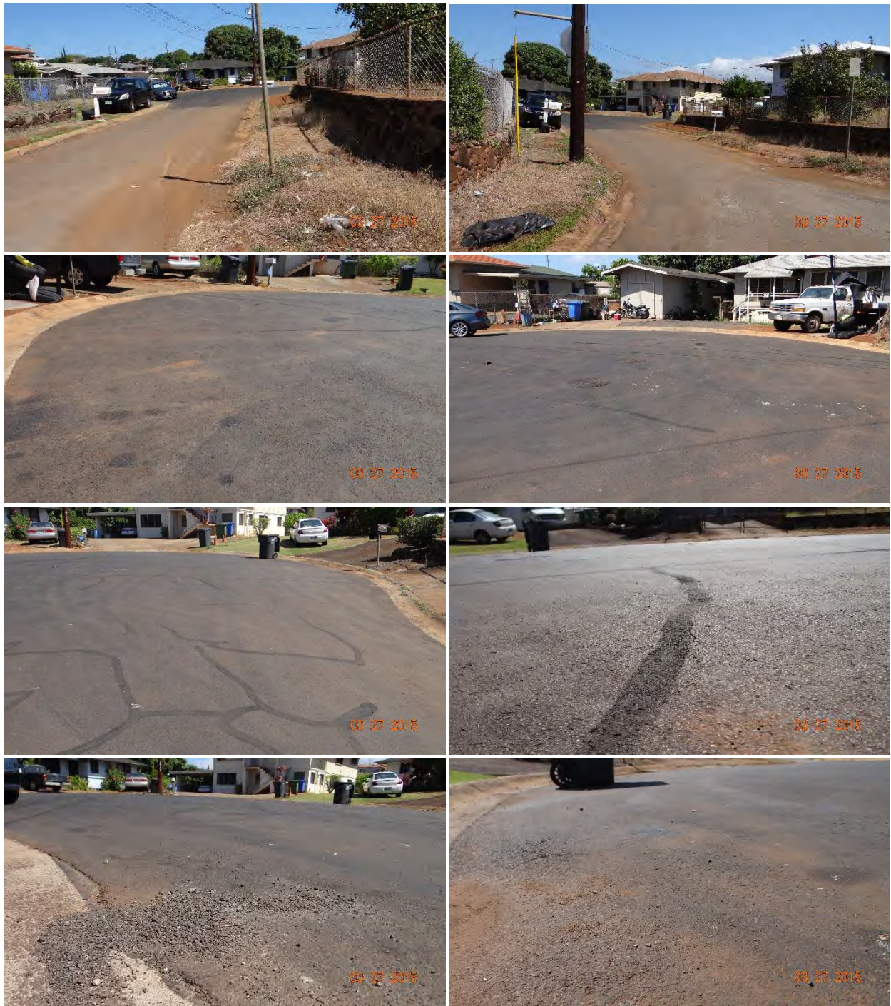
Figure C-99 Condition of the section on Hoolawa Place, treated with Plasti-Pave, on 3/27/2015.
