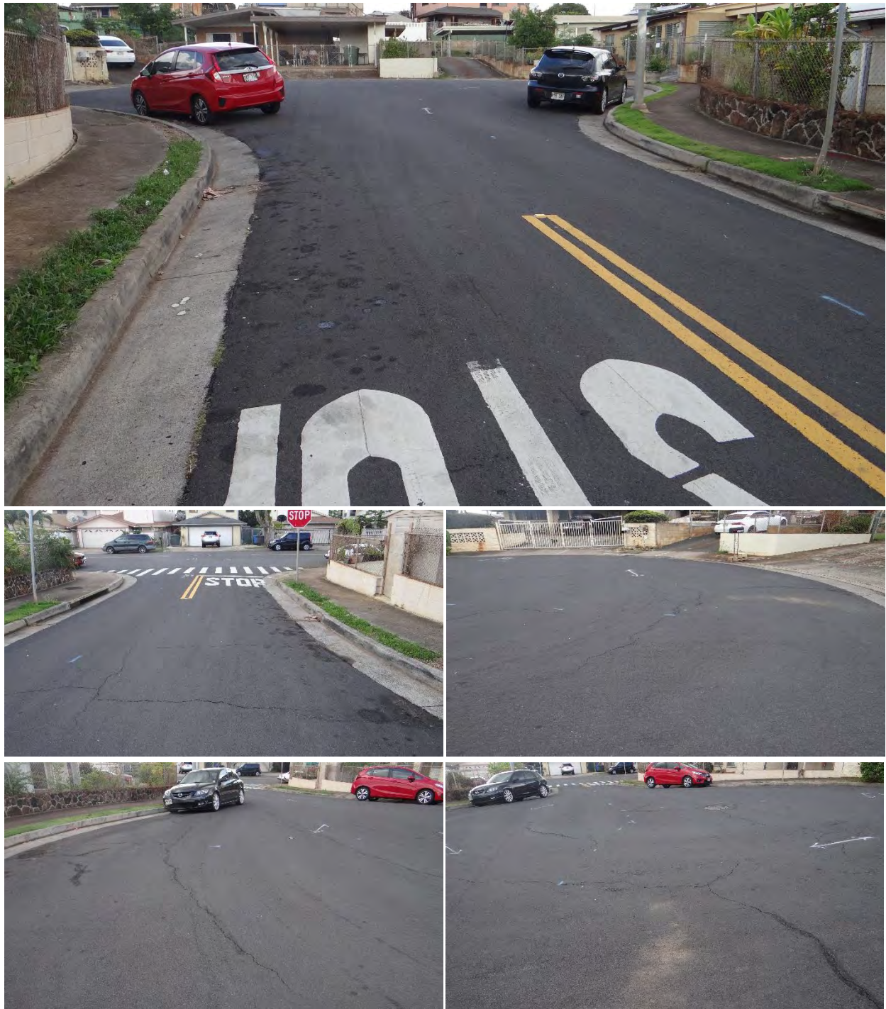
Figure C-158 Condition of the section on Hapapa Place, treated with Slurry Seal by Alakona Corp., on 2/7/2018.
