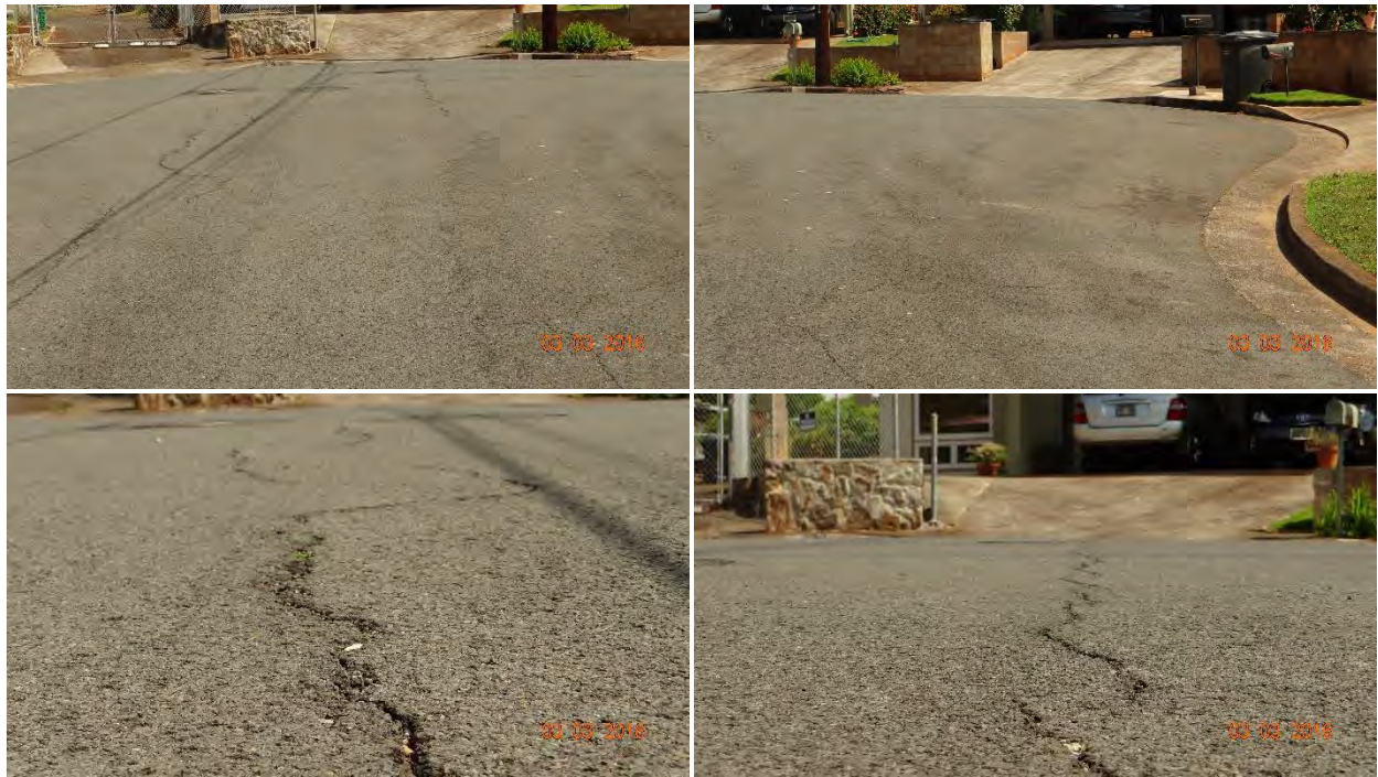
Figure C-96 Condition of the control section on Kaumoli Street on 3/3/2016.
