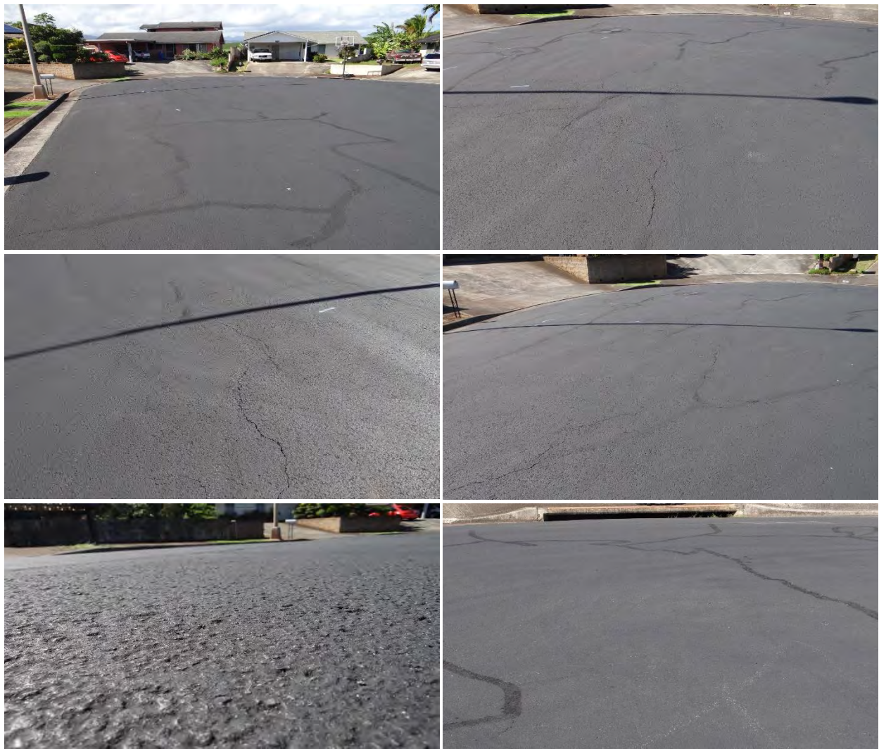
Figure C-115 Condition of the section on Kalauipo Place, treated with MasterSeal™ Ready to Use, on 12/14/2016.
