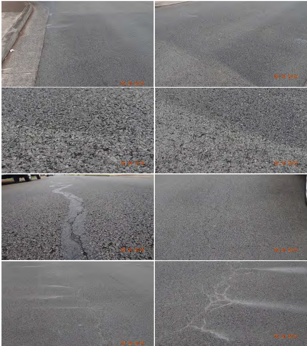
Figure C-57 Condition of Kaweloka Street section 1, treated with Plasti-Pave, on 5/24/2019.
