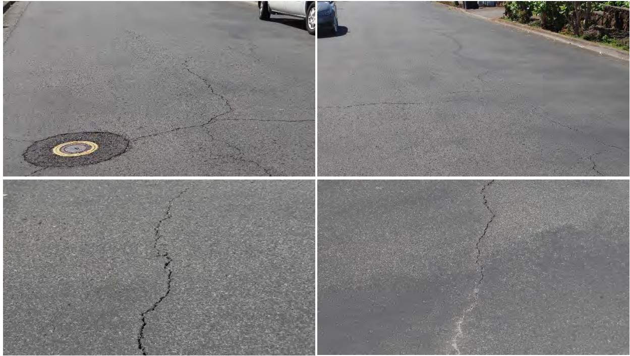
Figure C-93 Condition of section 5 on Kaweloka Street, treated with CarbonSeal-HF, on 1/26/2018.
