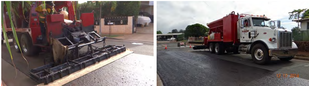
Figure 3-28 Slurry seal application.
