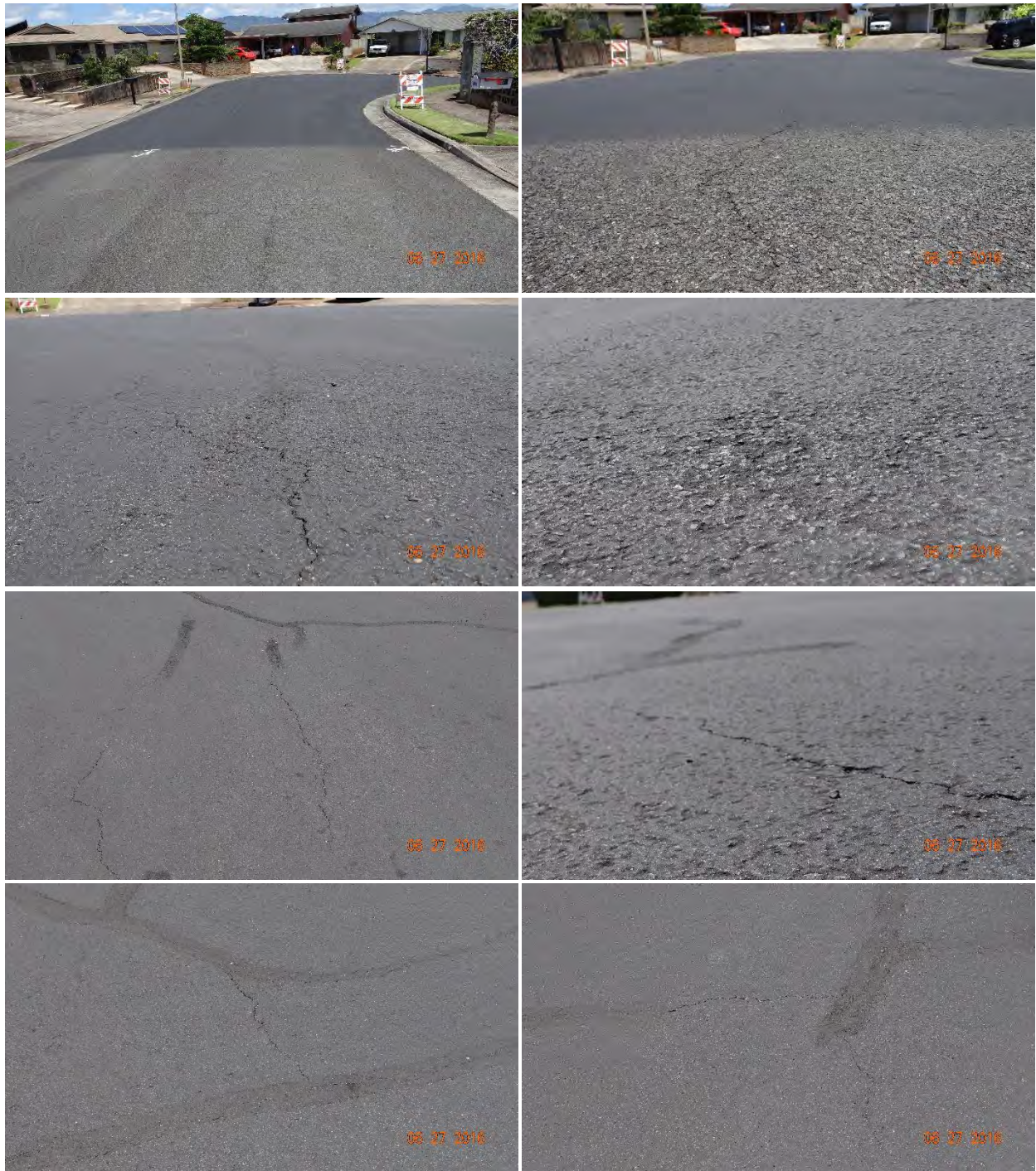
Figure C-114 Condition of the section on Kalauipo Place, treated with MasterSeal™ Ready to Use, on 6/27/2016.
