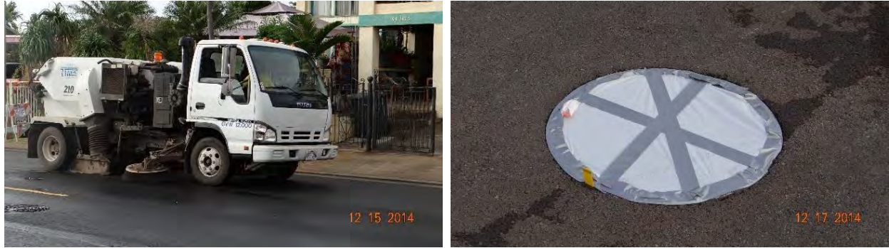
Figure 3-27 Aggregate sweeping (left) and manhole cover (right).
