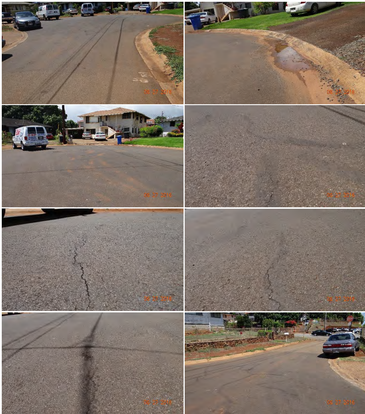
Figure C-101 Condition of the section on Hoolawa Place, treated with Plasti-Pave, on 6/27/2016.
