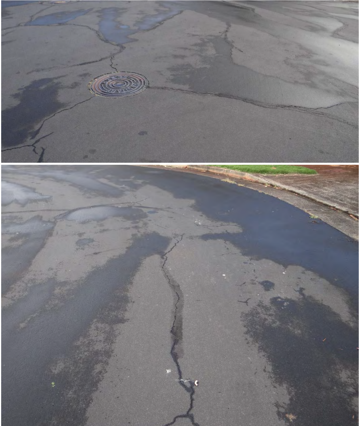
Figure C-108 Condition of the section on Kanihi Street, treated with Liquid Road, on 12/13/2016.
