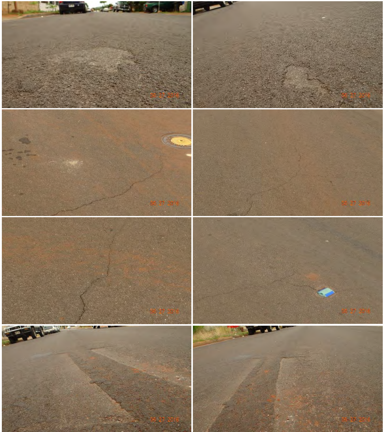
Figure C-142 Condition of the section on Hulahe Street, treated with Slurry Seal by Alakona Corp., on 6/27/2016.
