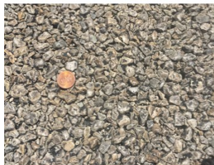
Location: Brownwood Right Wheel Path Mix Design: Dense Graded Type D
