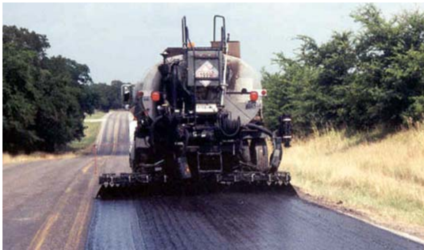
Figure 1.8: Application of Fog Seal (TxDOT, 2010)
