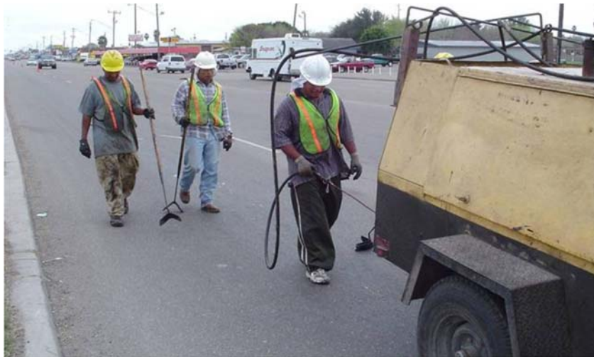
Figure 1.2: Application of Crack Sealing (Sims 2016)
