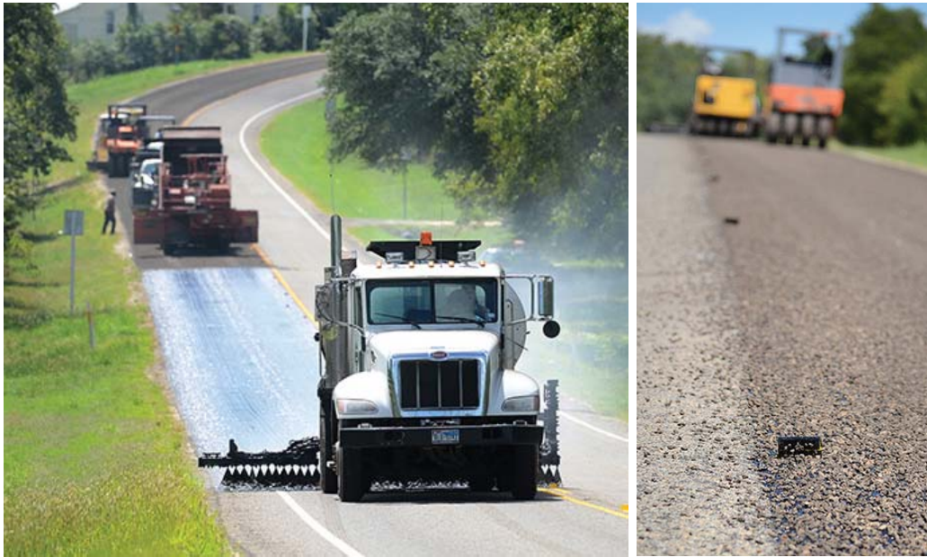
Figure 1.3: Application of seal coat (left) and rolling operation (right) (TTI, 2015)
