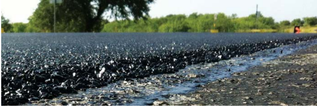
Figure 1.5: Layer of Thin Hot-mix Overlay (TTI, 2012)
