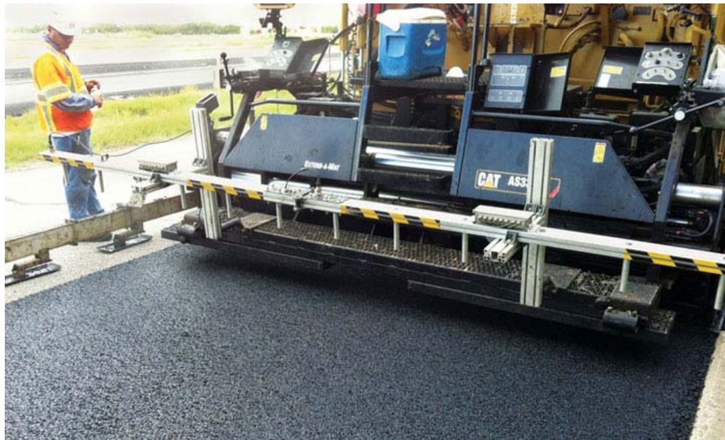
Figure 1.6: Application of Thin Hot-mix Overlay (TTI, 2012)
