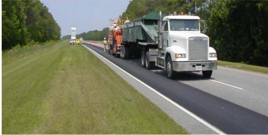
Figure 1.7: Application of Microsurface (Sims 2016)
